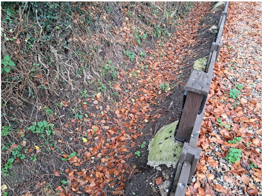
Figure 4 – New Bollard and kickboard.
