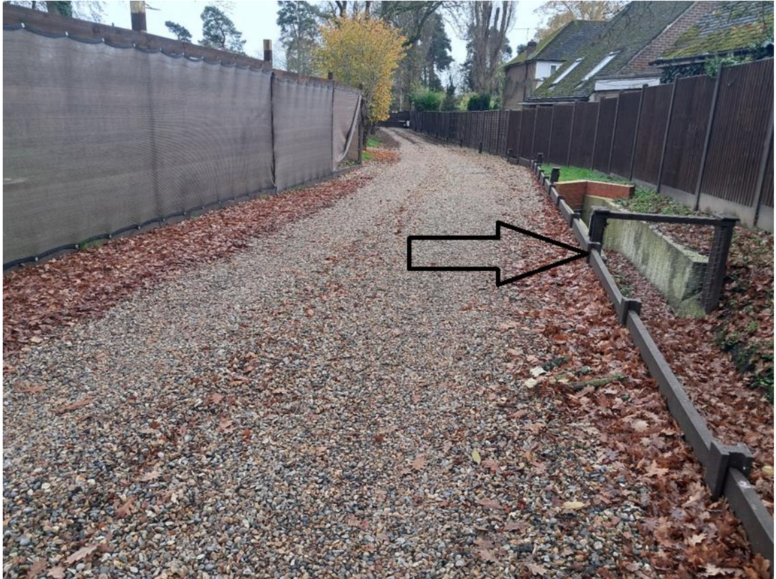
Figure 9 – Retaining wall & culvert at the southern end of the ditch.
