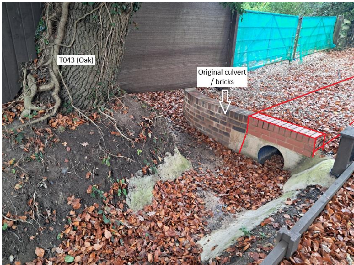
Figure 12 – New culvert (shown in red) at the northern end of the ditch.
