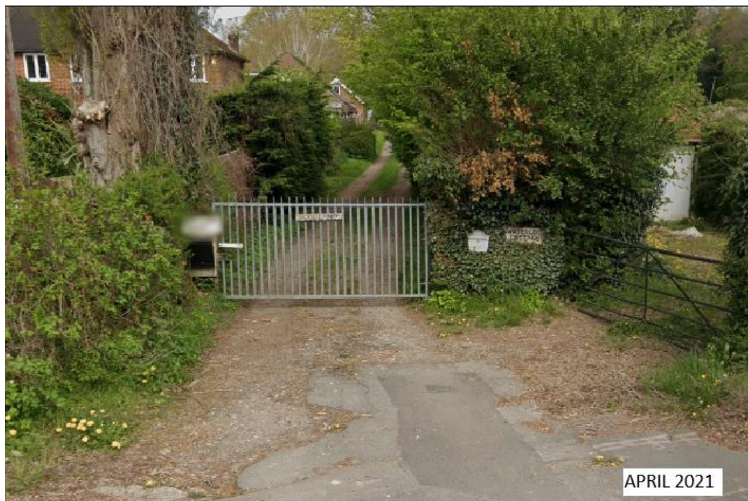
Figure 1 – Google Street View image of the access driveway from April 2021 – prior to resurfacing works
