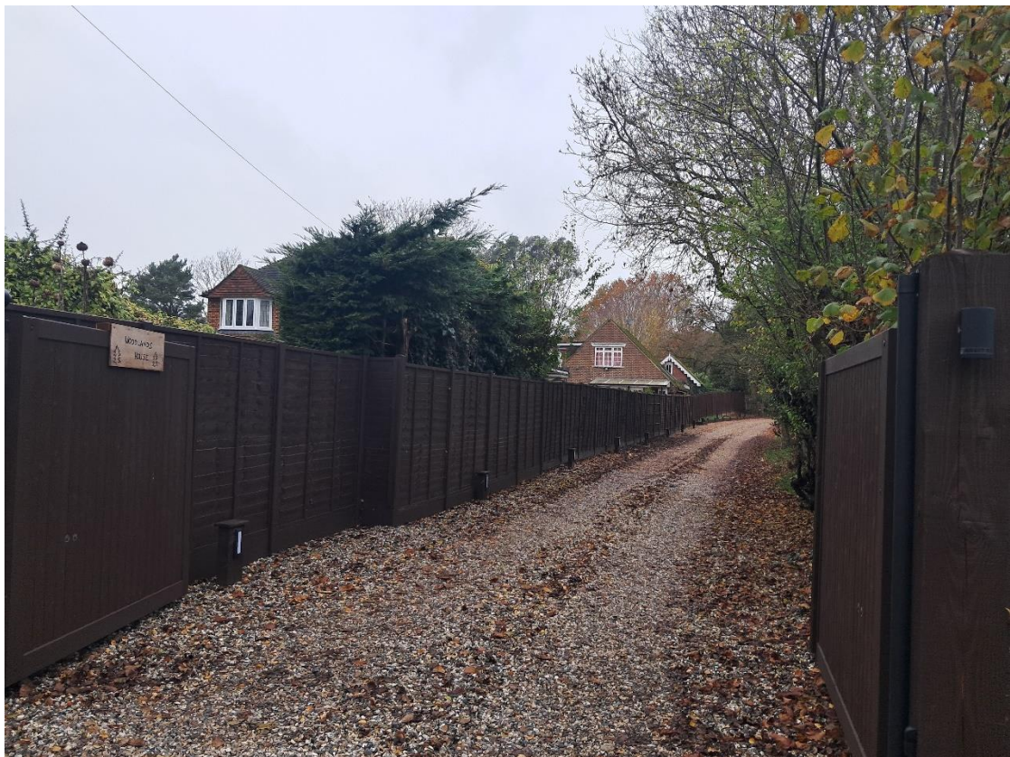
Figure 3 – Photo of the access driveway from November 2024 with new aesthetic stone / gravel surface.
