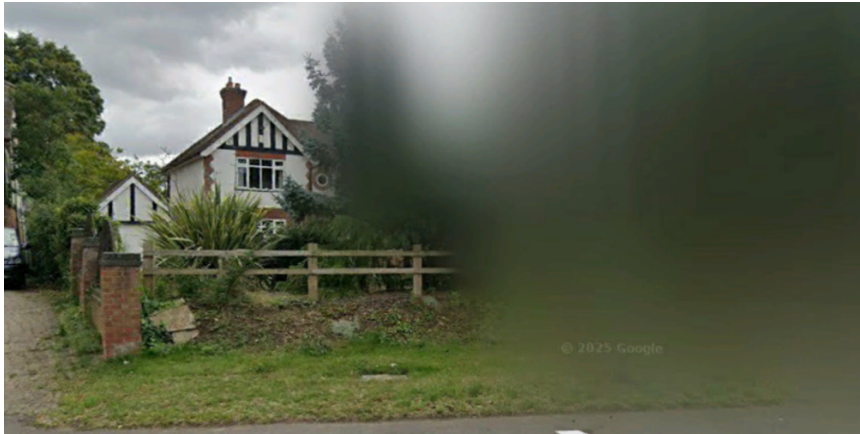
Figure 2 2024 Google Street view shows a section of front boundary at 8 Pitts Lane
