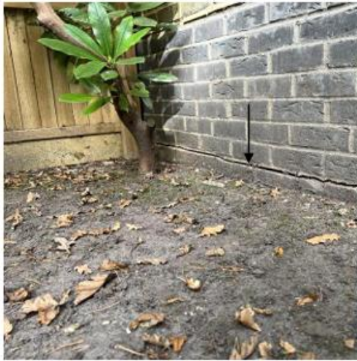
Right flank looking towards front
