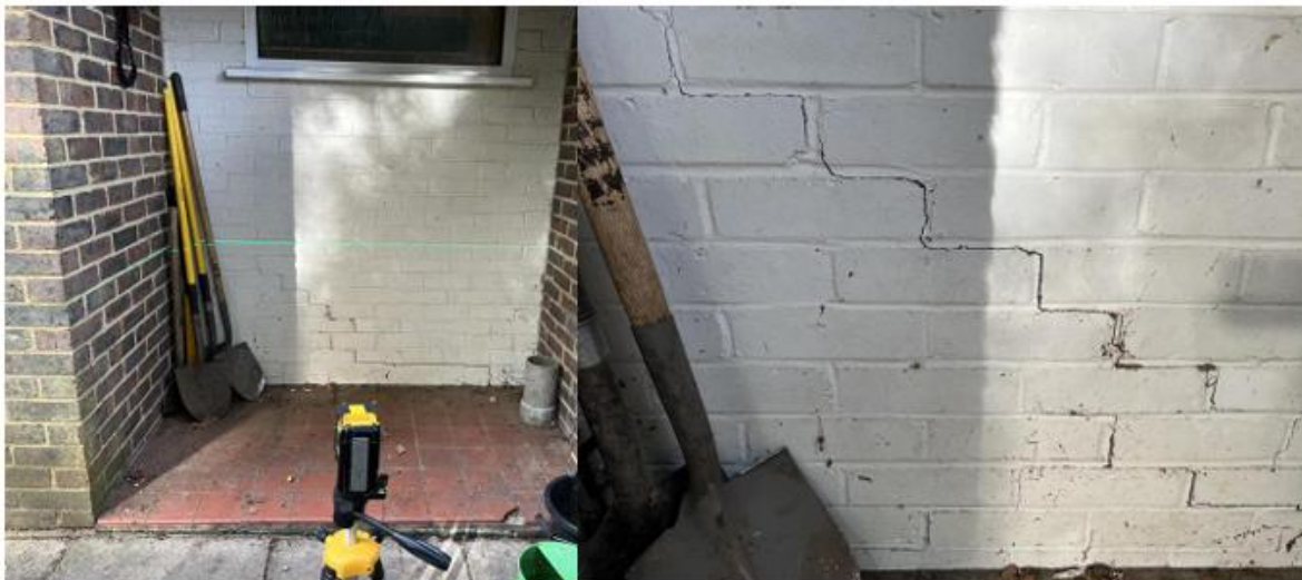
Garage rear wall – level brickwork
