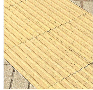
5 Cordouroy paving at tops and bases of ramps and steps
