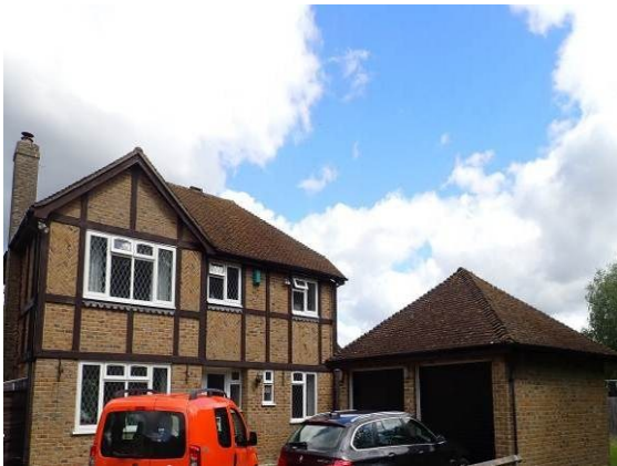
Photograph 1. Front of house and garage viewed from southwest.
