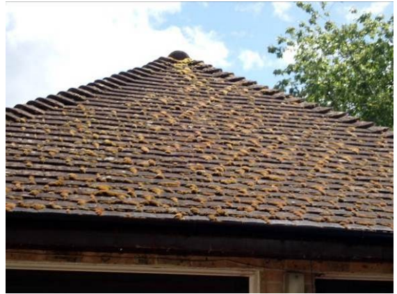
Photograph 12. The tightly fitted, flat tiles and hips.
