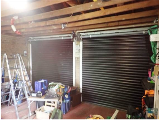
Photograph 20. The interior of the garage open to the void above.
