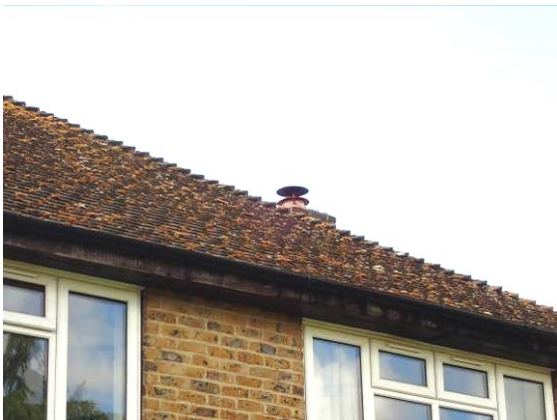
Photograph 3. Flat, tightly fitted roof tiles and fully intact ridge and hip mortar (rear elevation).
