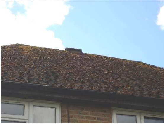
Photograph 5. Ridge vent (rear elevation).
