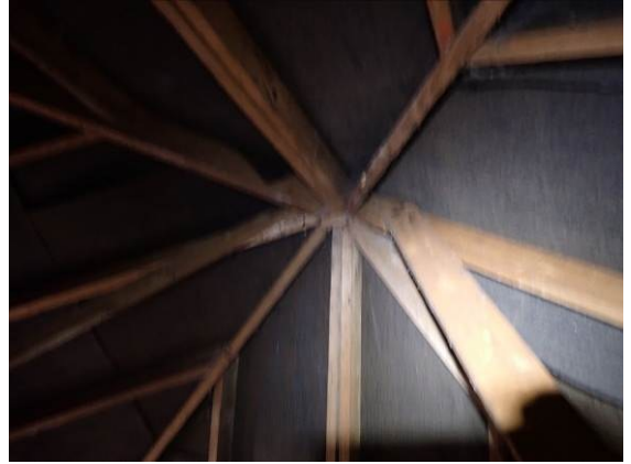
Photograph 21. Cobwebbed timbers and intact bitumen felt at the apex.
