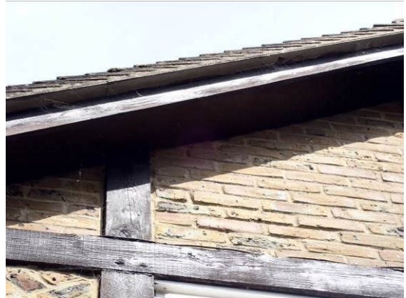
Photograph 8. Tightly fitted soffits (front gable).
