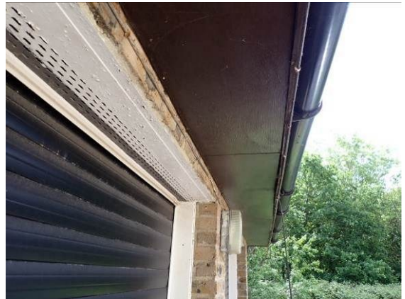
Photograph 13. Tightly fitted soffits.
