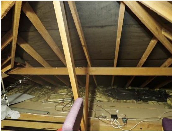
Photograph 16. Intact, tightly fitted bitumen felt.
