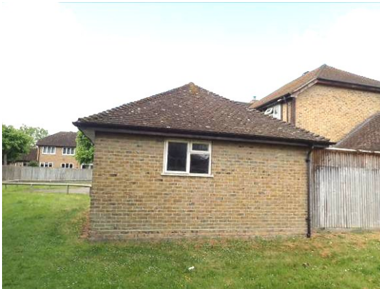
Photograph 13. The garage viewed from the rear (east)
