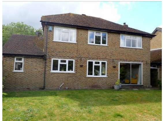
Photograph 2. Rear of property viewed from northeast showing single storey roof to the rear of the garage.
