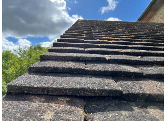
Photograph 6. Slightly raised verge tiles on rear of single storey roof showing no evidence of bats during an endoscopic inspection.
