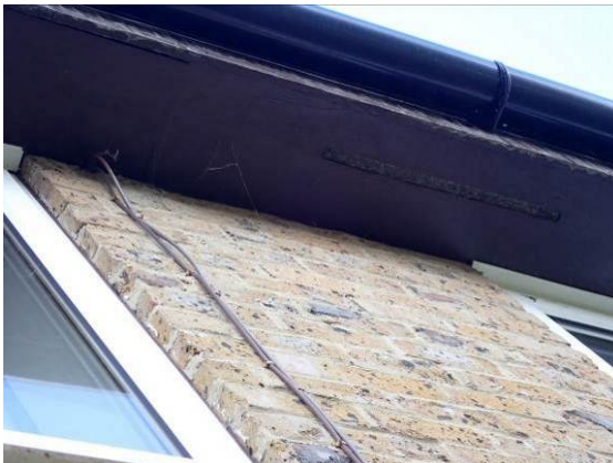
Photograph 9. Tightly fitted soffits (front elevation).
