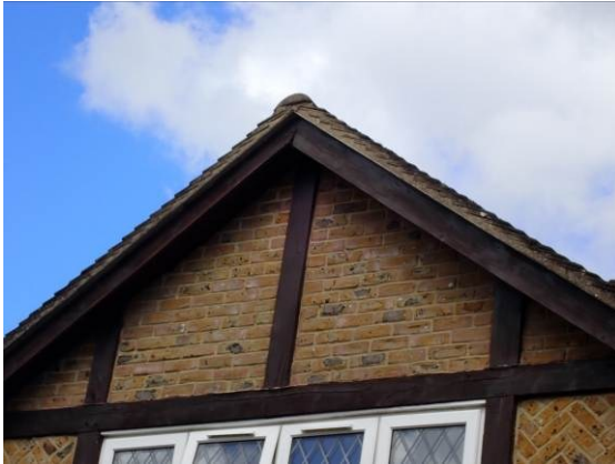
Photograph 7. Intact verge mortar on front gable.
