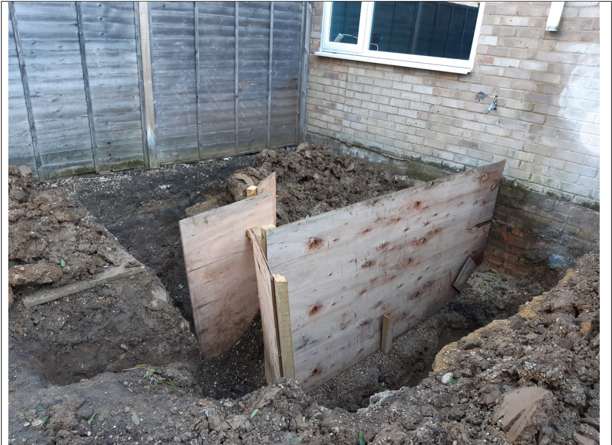
Figure 2: Enforcement Case Officer photograph of rear extension (29/09/2020)
