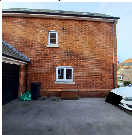
Figure 2- No.16 window & driveway
