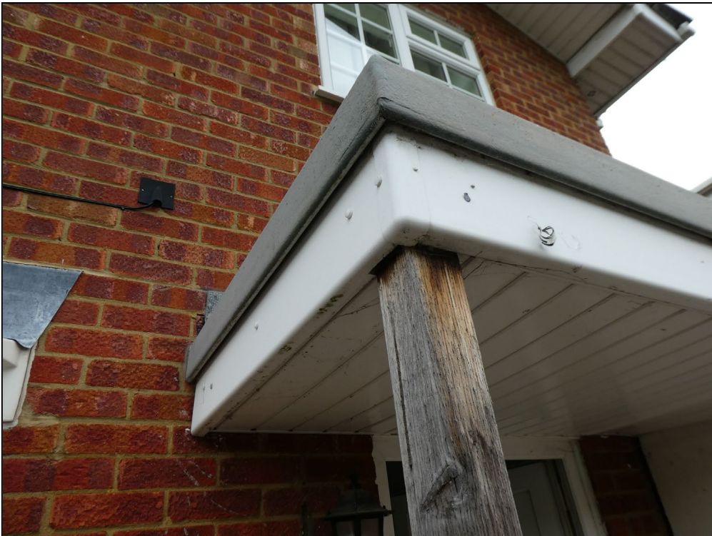
Figure 8. The flat roof over the front porch. 10 Russell Way, Winnersh. 10.09.24
