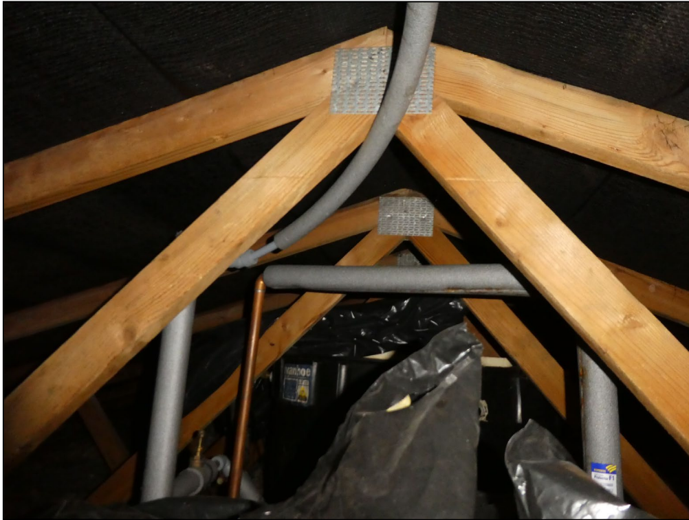
Figure 12. Example of bitumen lining. 10 Russell Way, Winnersh. 10.09.24
