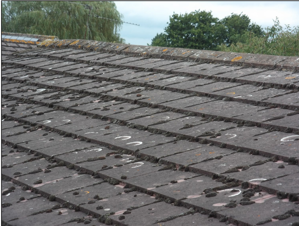
Figure 4. Example of roof tiles. 10 Russell Way, Winnersh. 10.09.24
