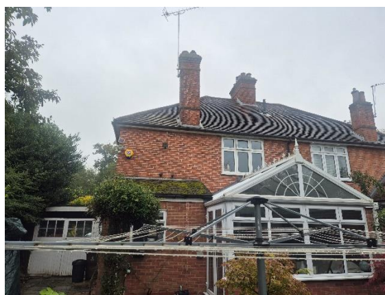
Photograph 4: Southern elevation of B1.
