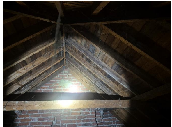
Photograph 8: Loft void of B1.
