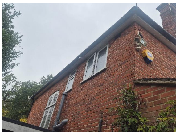
Photograph 3: Western elevation of B1.
