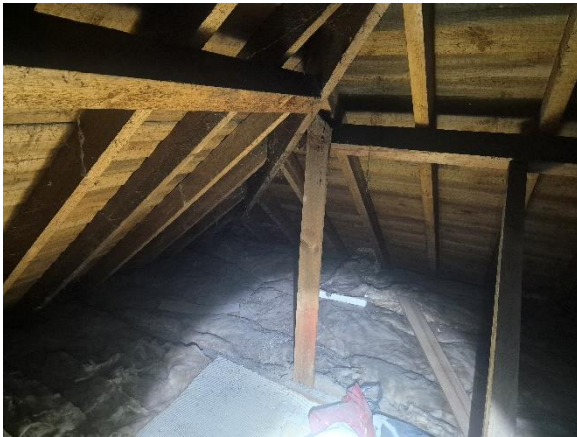
Photograph 7: Loft void of B1.
