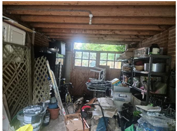
Photograph 10: Interior of the garage of B1.
