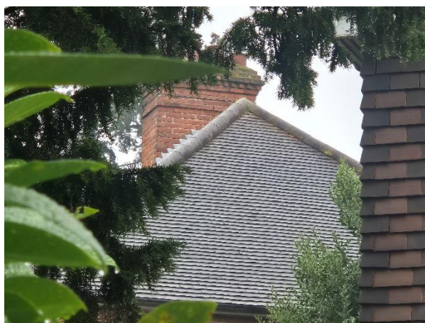
Photograph 14: Roof on the western elevation of B1.
