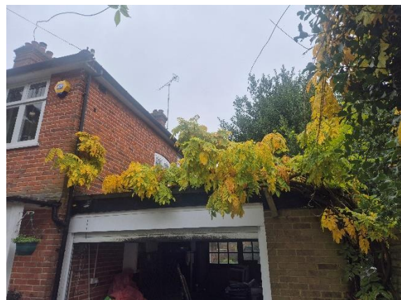
Photograph 2: Northern elevation of the attached garage of B1.
