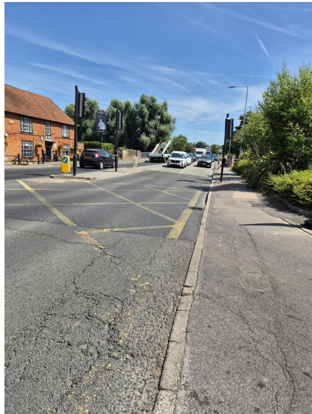
Taken from Entrance / exit from kerb position Person in blue top is standing at kerb line at 120m and is not visible because of curvature of road and bridge pilaster
