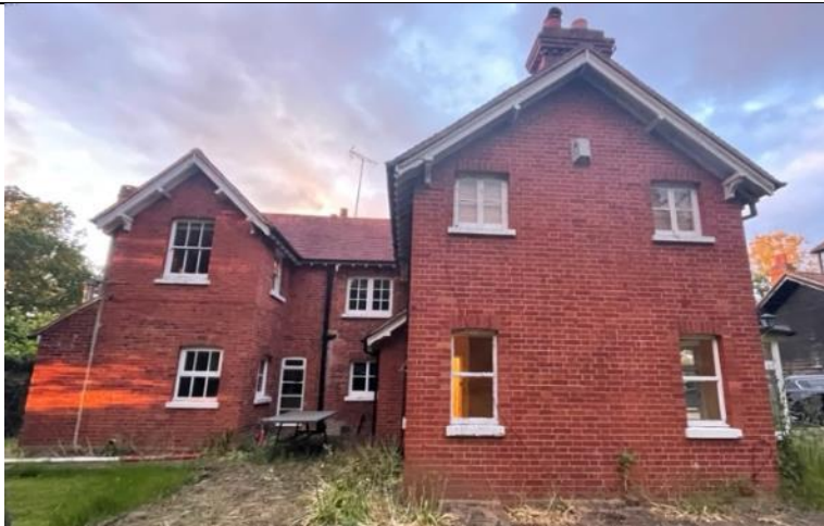
Figure 4: the south-western elevation of B2
