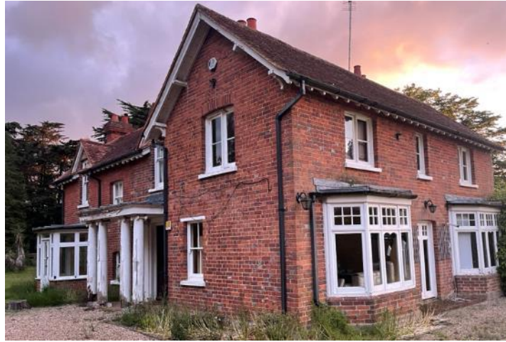
Figure 2: the north-eastern and south-eastern elevations of B2
