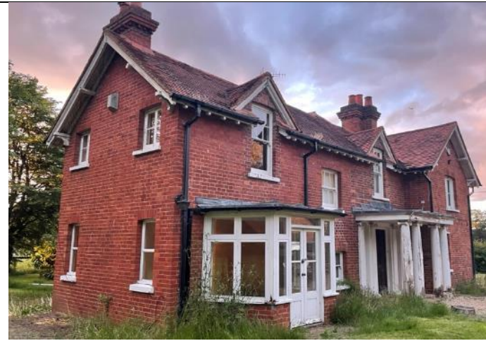
Figure 5: the south-eastern elevation of B2
