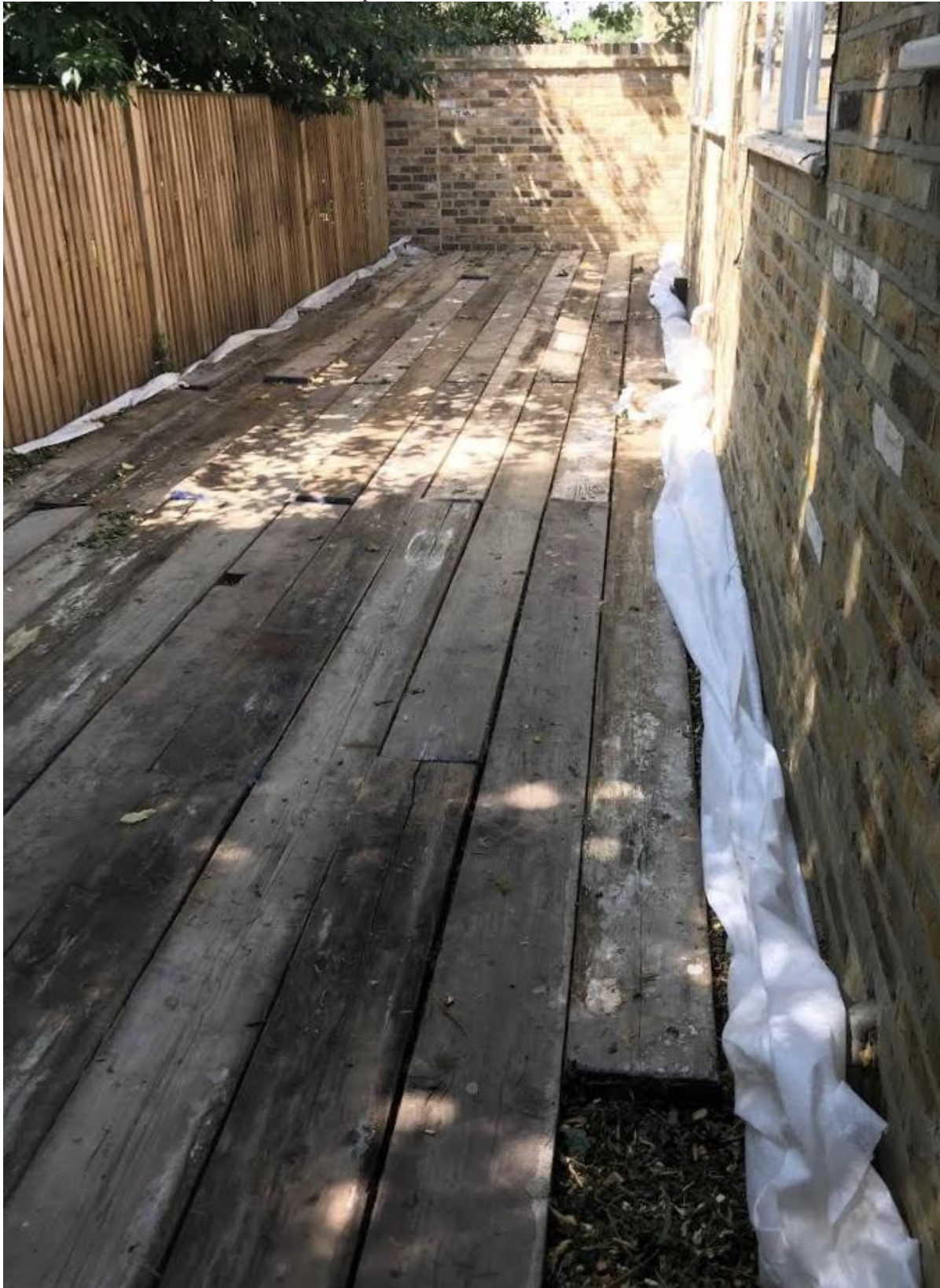
Photo 1. Scaffold boards placed on woodchip
