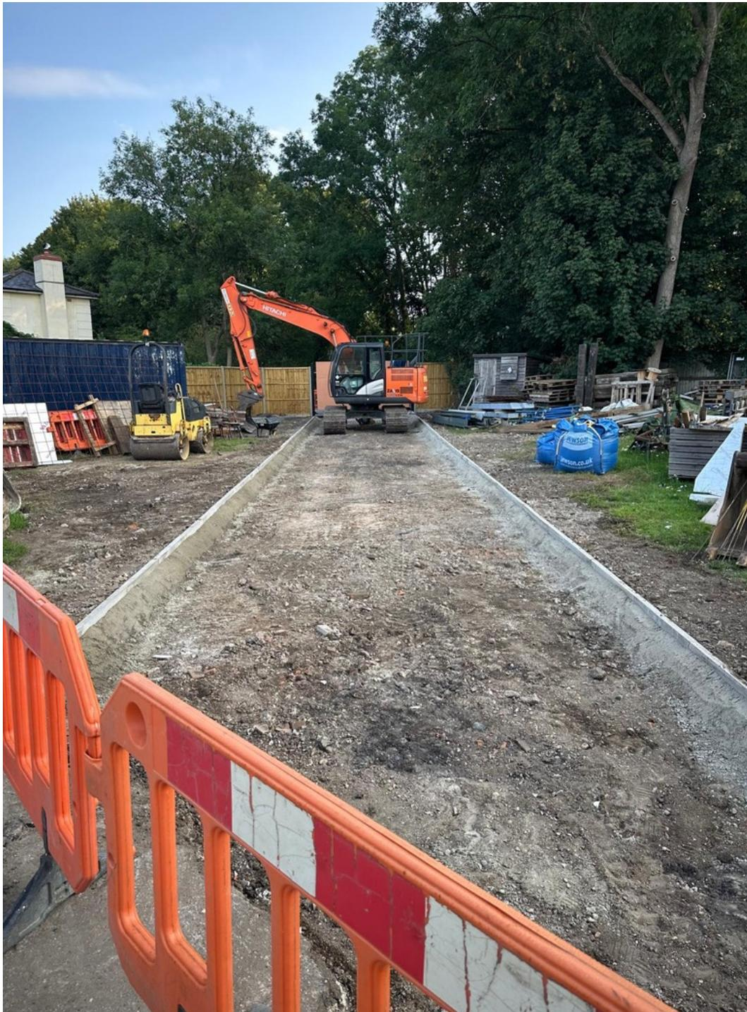
The roadway is constructed with layers of compacted crushed rock to form a robust but permeable surface, restrained at the sides with concrete edges. The finished surface is at the same level as the existing ground so it will have no impact on flood water storage capacity nor increase flood risk elsewhere.
