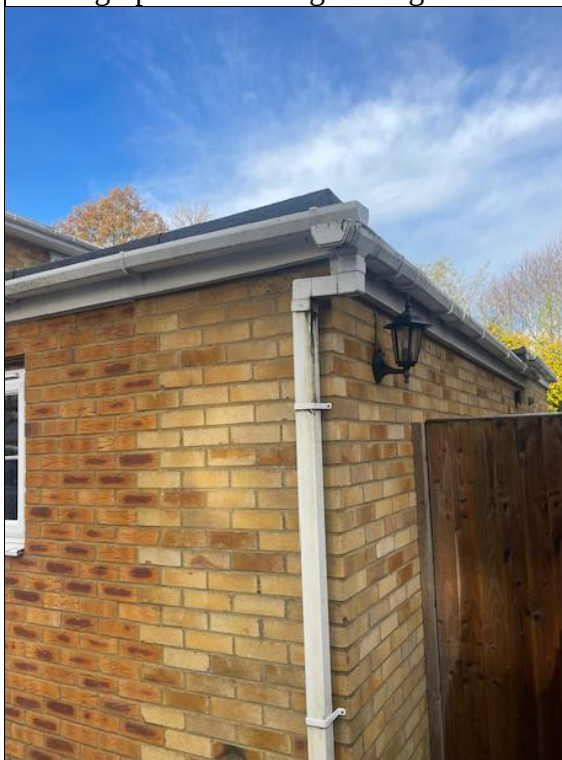
Photograph 15: Side of flat-roofed section of house.
