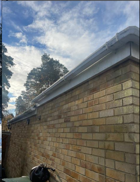
Photograph 12: Single-storey section of house.
