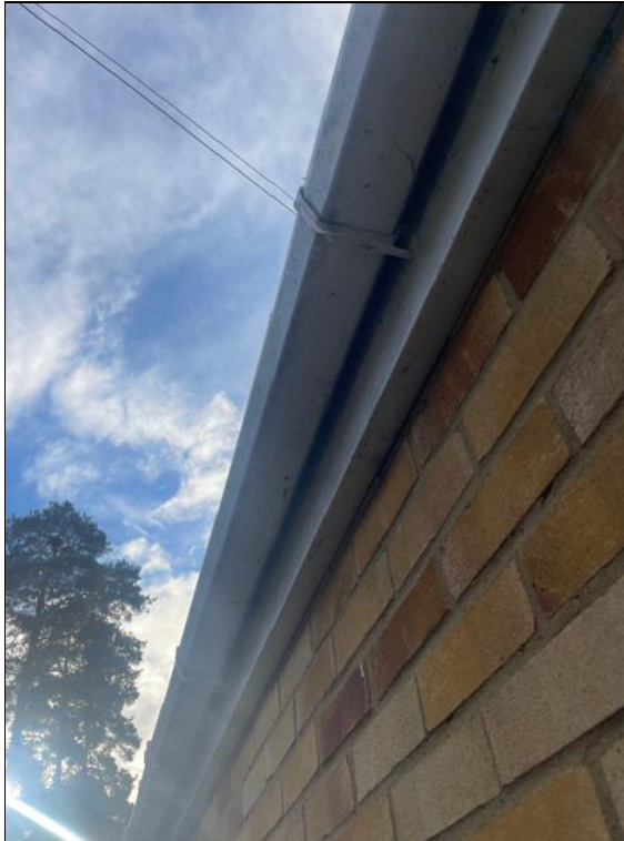
Photograph 13: uPVC guttering.
