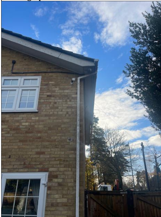
Photograph 7: Soffits in good condition.
