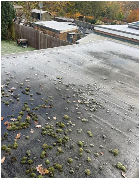
Photograph 1: Flat-roofed, single storey extension.
