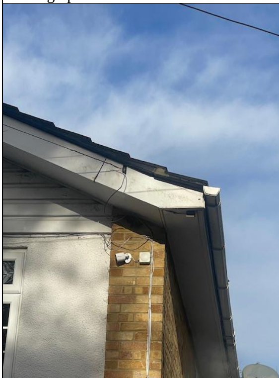
Photograph 19: Soffits in good condition.
