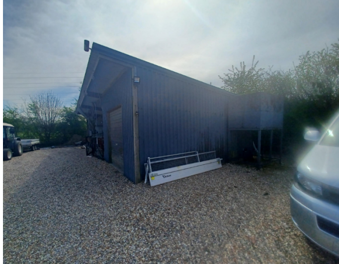
Figure 4 - Site visit photo taken on 08/04/2025 showing the subject building and extent of vegetation of the along the south-western side boundary.
