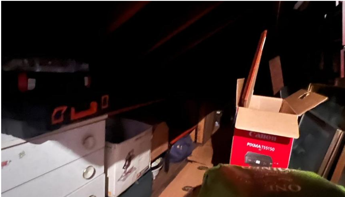
Plate 7: Image of the loft void within B1 .
