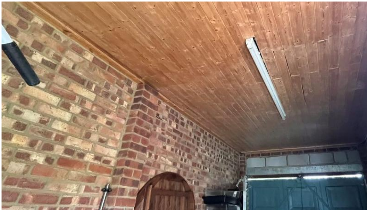
Plate 9: Image of the internal of the garage section of B1 .
