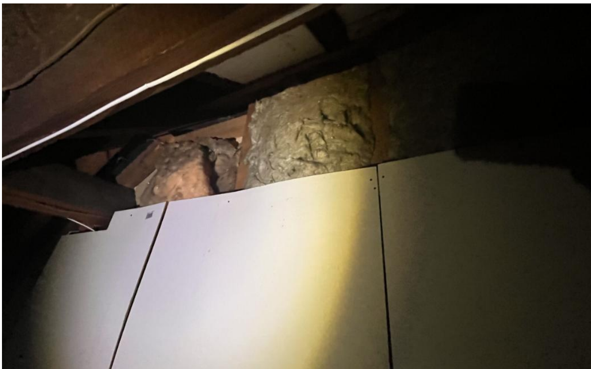
Plate 6: Image showing the flooring in the loft space.
