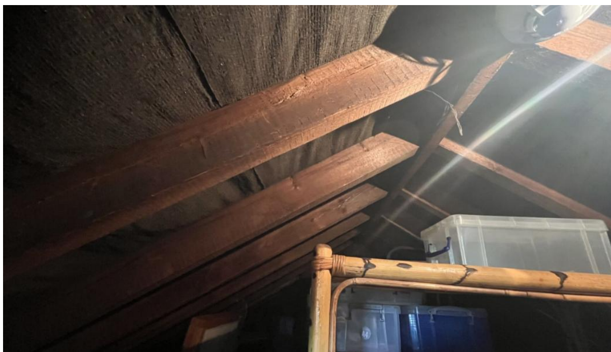
Plate 7: Image showing the timber beams in the loft roof space.
