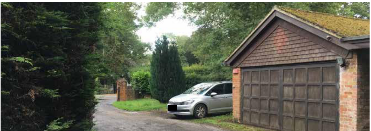
5. Existing access and double garage
