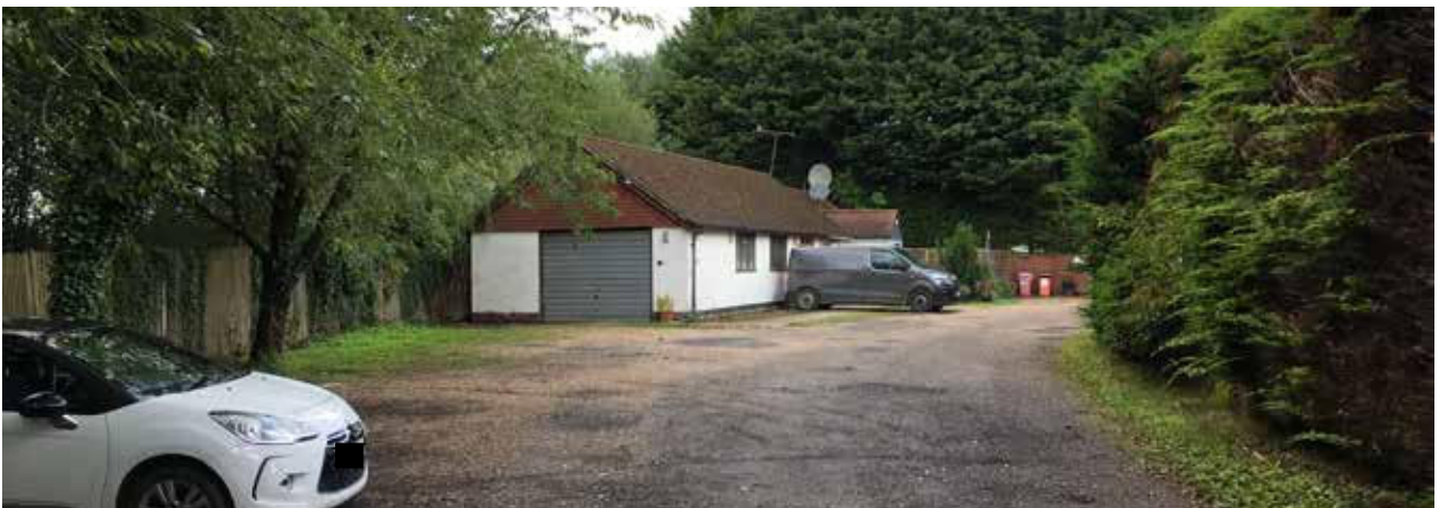
3. South-western edge of site
