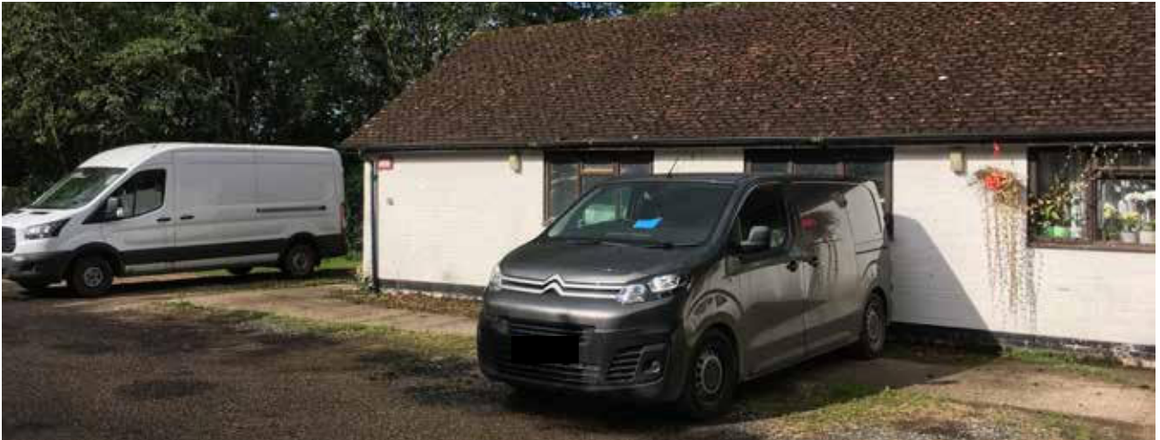
4. South-western edge of site
