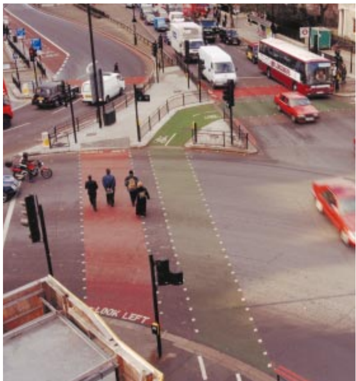
Hyde Park Corner — After: new at-grade crossing for pedestrians.
