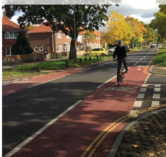
Figure 6.21: Centre line removal, Norwich
