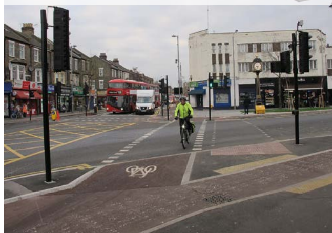
Figure 10.26: Circulating Cycle Stage Junction, Waltham Forest
