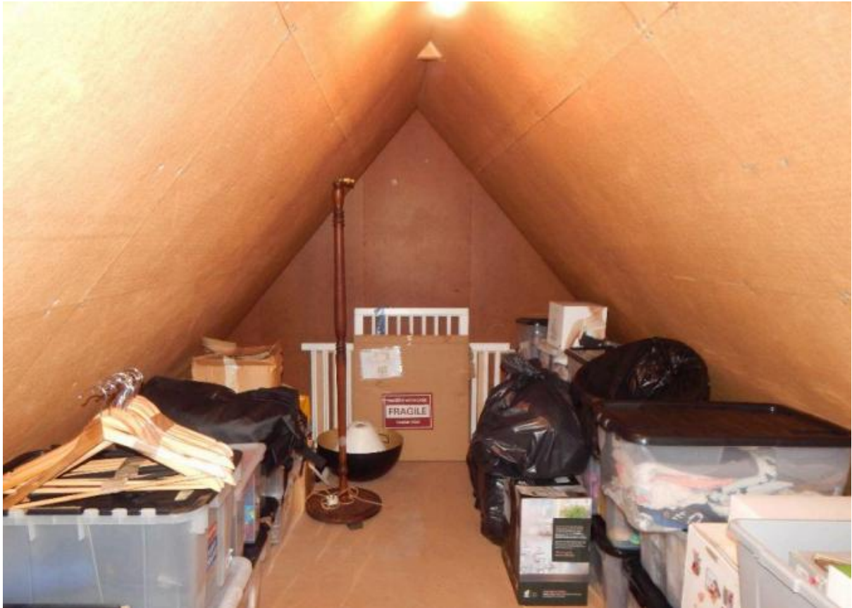
Image 9 – Internal view within the vaulted section of the property
