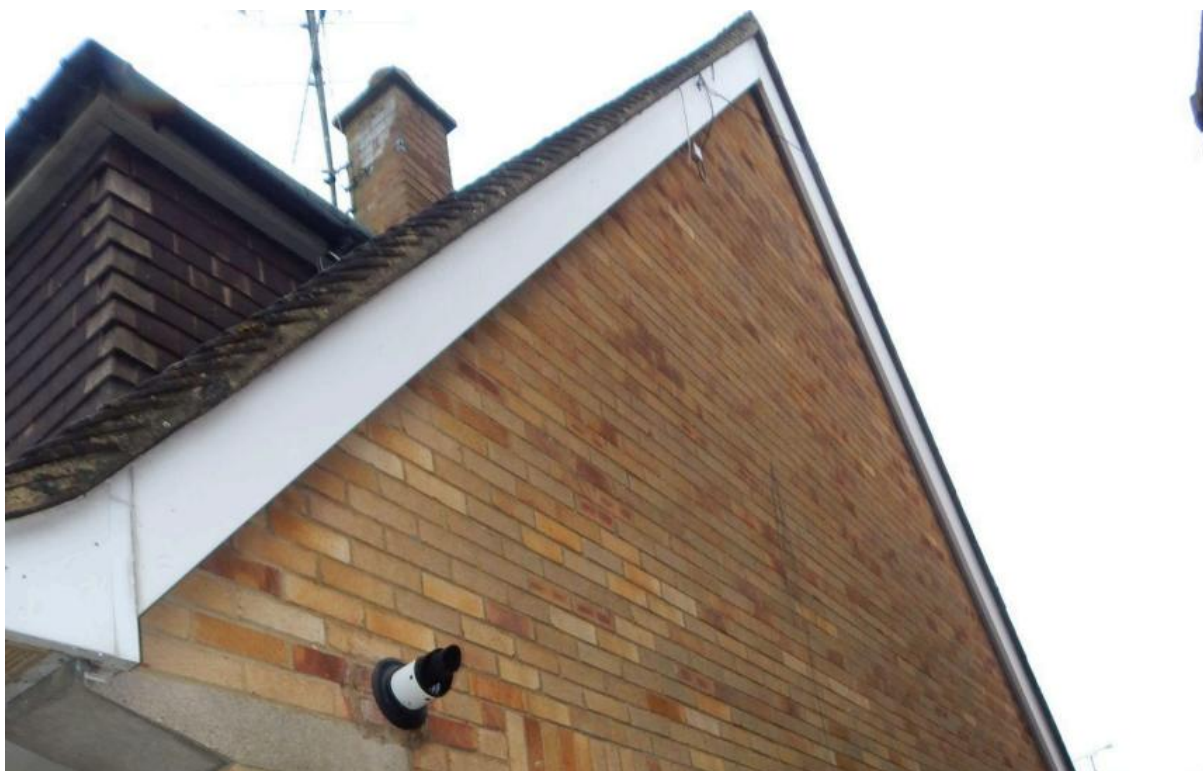
Image 6 – West facing elevation of the property
