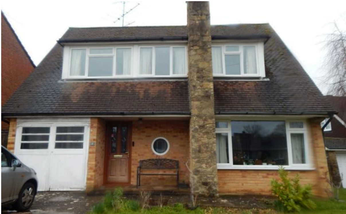
Image 1 – South facing elevation of the property
