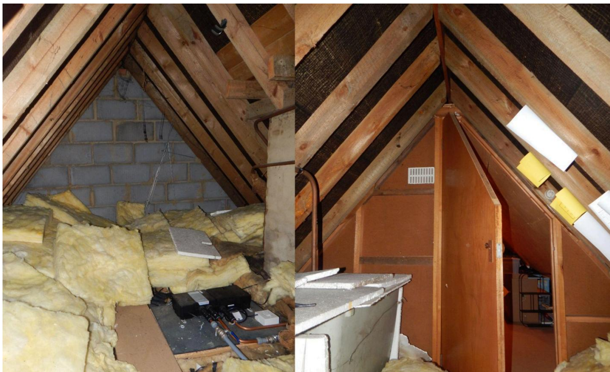
Image 8 – Internal views from within the accessible roof void spaces of the property
