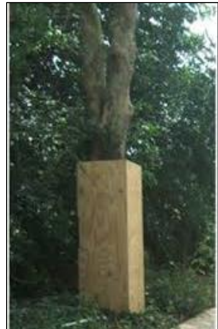
Plate 4: Example of plywood hoarding used as tree protection. ©Google.
