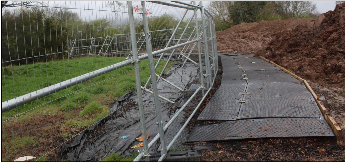
Plate 3: An example of temporary ground protection laid up against the tree protection fencing. This protects the RPA whilst also providing adequate space between the fencing and the development footprint.
