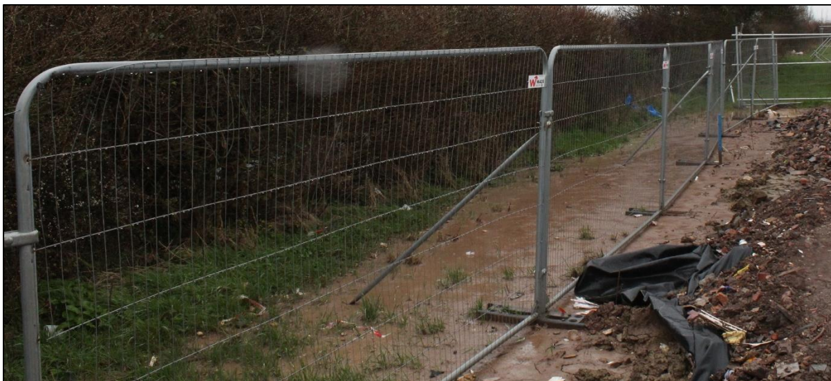
Plate 2: An example of the alternative tree protection fencing specification.
