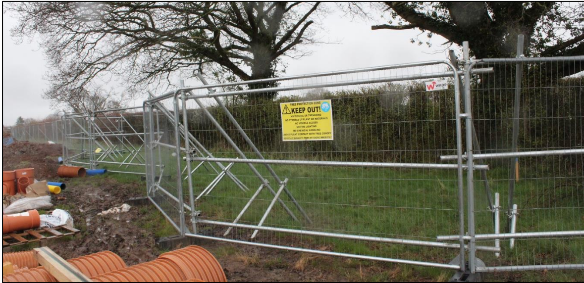
Plate 1: An example of the default tree protection fencing specification.
