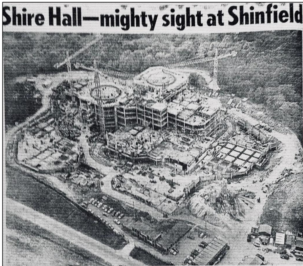
Photograph 2. Shire Hall construction 7
