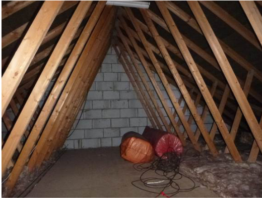
Photograph 7. Roof void with trussed rafters.
