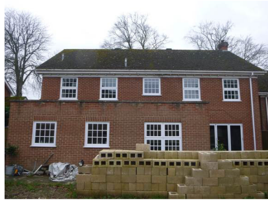
Photograph 2. Rear of property viewed from south.
