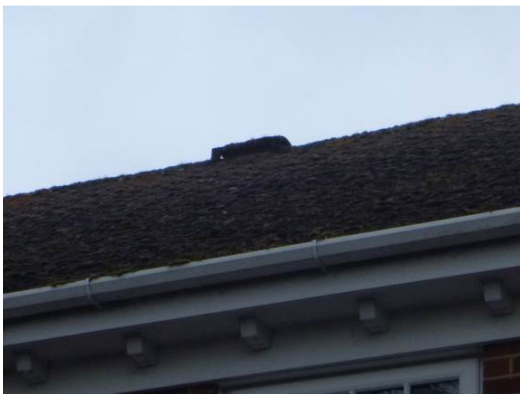
Photograph 5. uPVC soffit tight to brickwork throughout.
