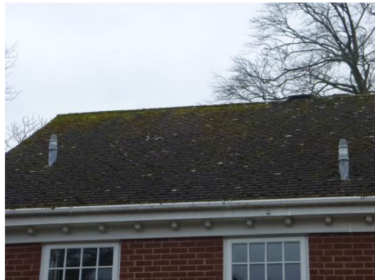
Photograph 4. Ridge tiles and mortar intact throughout.
