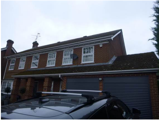
Photograph 1. Front of property viewed from north.
