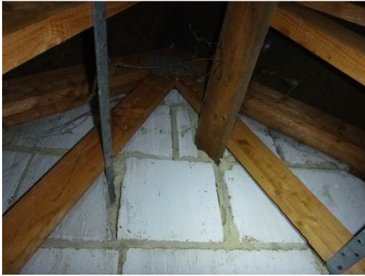
Photograph 11. Blockwork gables filled around rafter gaps.
