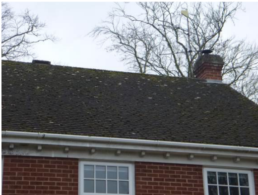
Photograph 3. Flat roof tiles intact throughout.
