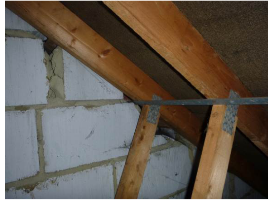
Photograph 12. Blockwork gables filled around rafter gaps.
