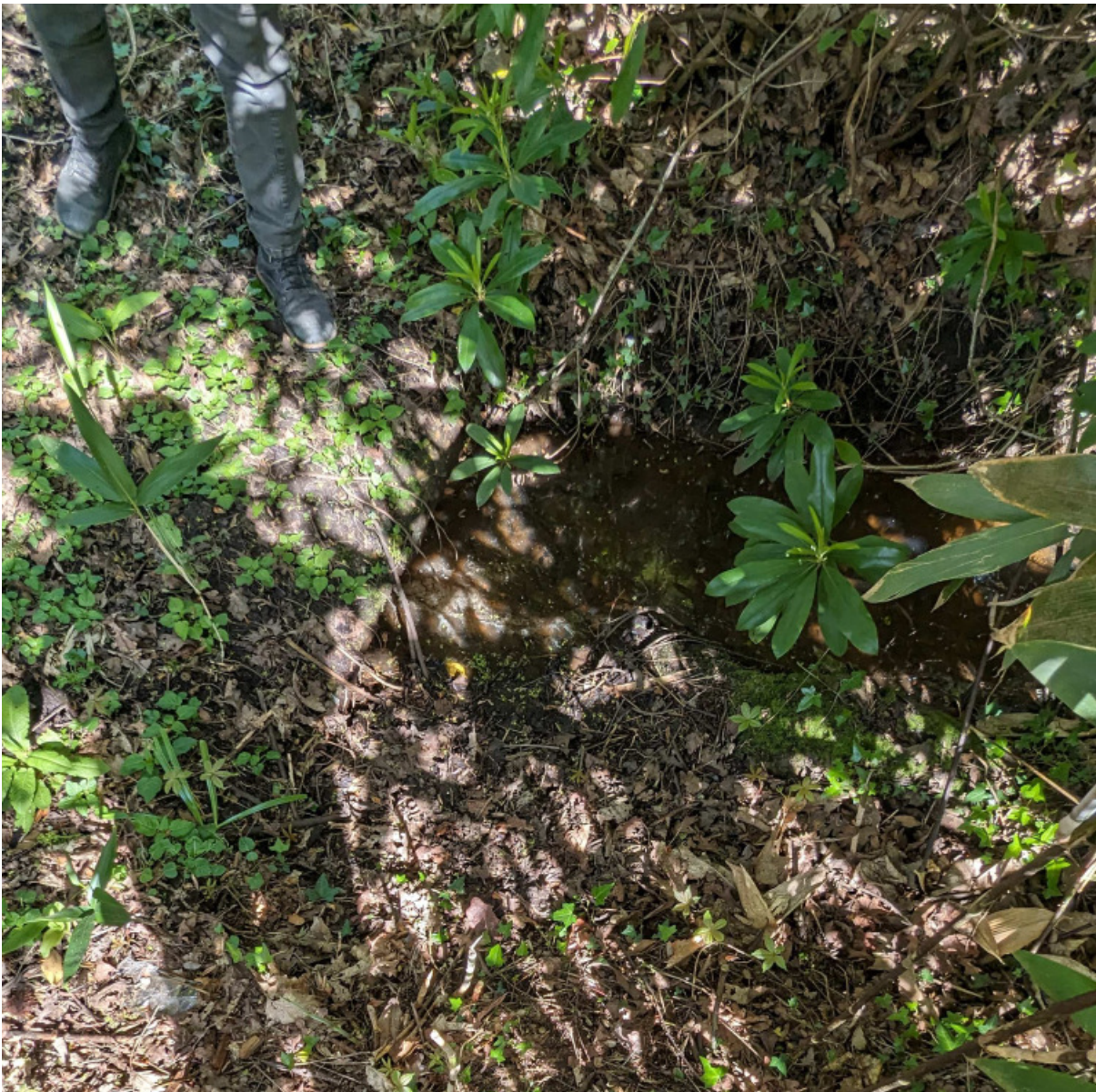
Showing small 'bridge' over the ditch and the water in the ditch
