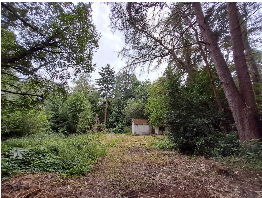
Photo 4 – Access to Old Louma Cottage.
