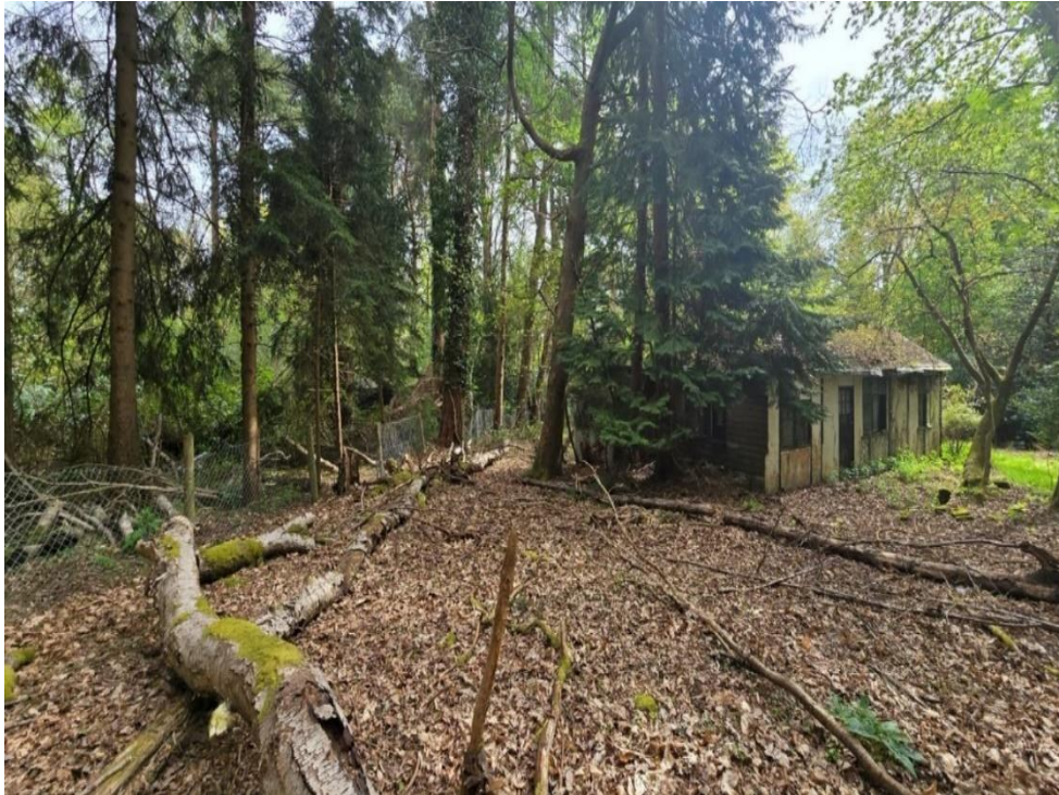
Plate 3: Image showing the north-west elevation of B1 .
