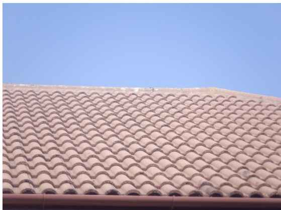
Photograph 3. Tightly fitted, interlocking concrete tiles (rear elevation).
