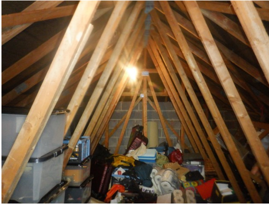
Photograph 11. Void of trussed construction.
