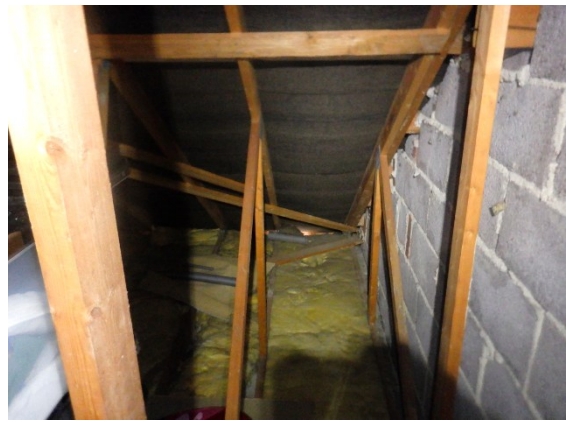
Photograph 13. Open eaves with access to the painted timber soffit.
