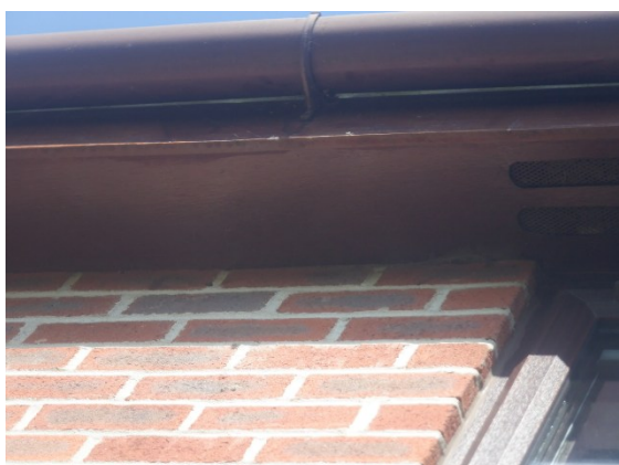
Photograph 9. Vented soffit sealed to brickwork (rear elevation).
