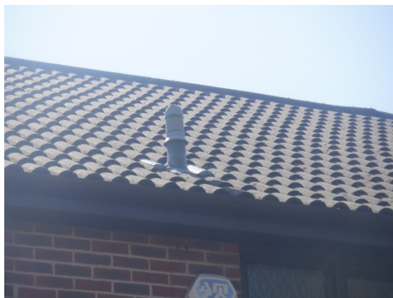
Photograph 7. Lead flashing flat around the base of the flue pipe (front elevation).
