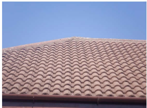
Photograph 4. Fully intact ridge and half-hip mortar (rear elevation).
