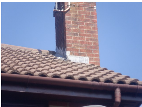
Photograph 6. Lead flashing flat around the base of the chimney (rear elevation).
