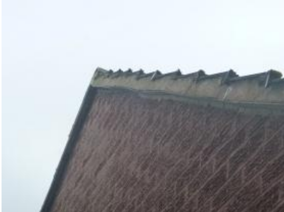
Photograph 7. Intact verge mortar along garage gable (northern elevation).
