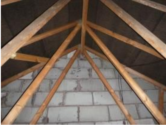
Photograph 14. Void of trussed construction (Roof void 1).
