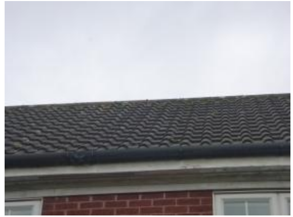
Photograph 6. Sealed roof tiles and ridge tiles along the second-storey (southern elevation).
