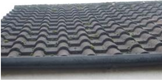
Photograph 5. Sealed roof tiles and ridge tiles across the garage (eastern elevation).
