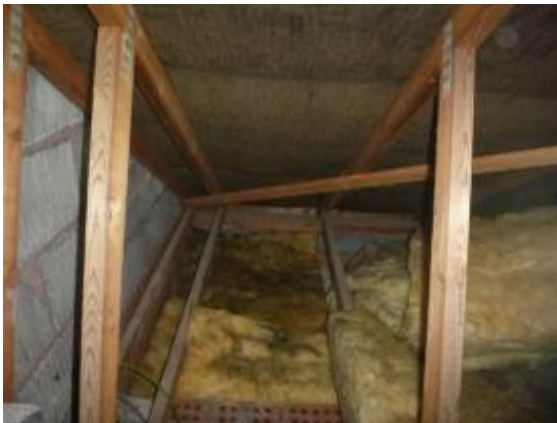
Photograph 15. Bitumen felt fully sealed (Roof void 1).
