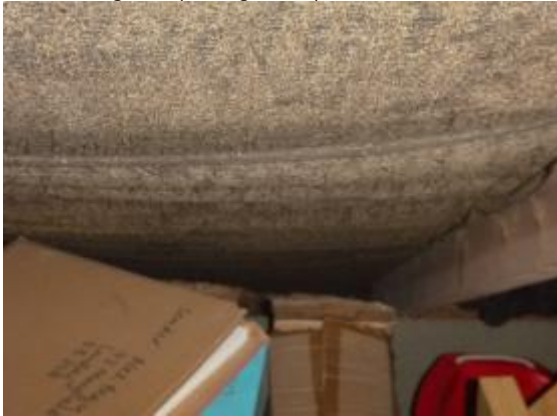
Photograph 21. Open eaves (Garage void).
