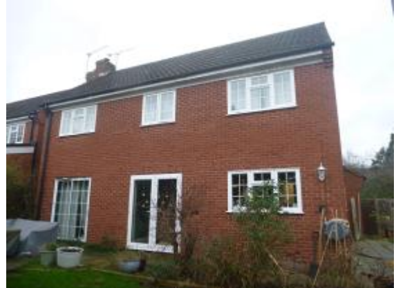
Photograph 2. Rear of property viewed from southeast..
