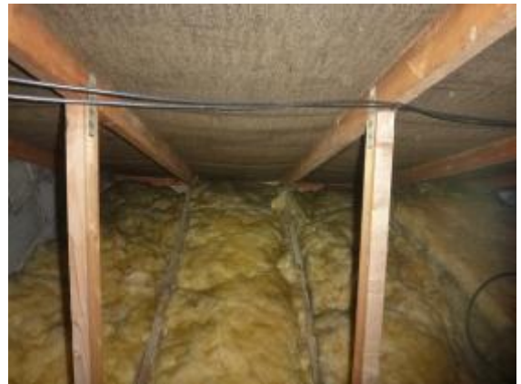
Photograph 16. Open eaves (Roof void 1).
