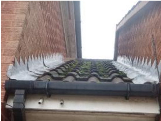
Photograph 11. Lead flashing sealed to brickwork and roof tiles (eastern elevation).
