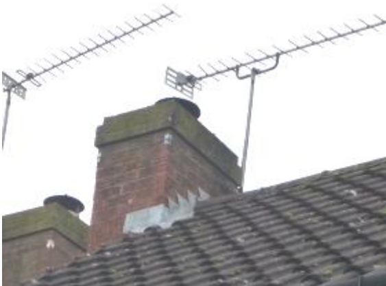
Photograph 9. Lead flashing sealed to brickwork chimney (rear elevation).
