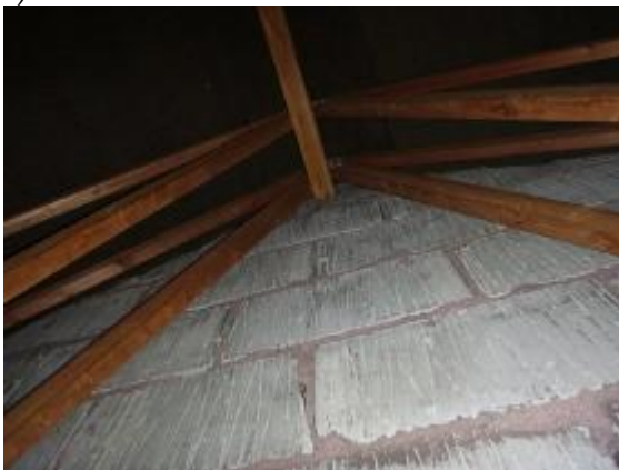
Photograph 17. Timbers sealed to south blockwork internal wall (Roof void 1).
