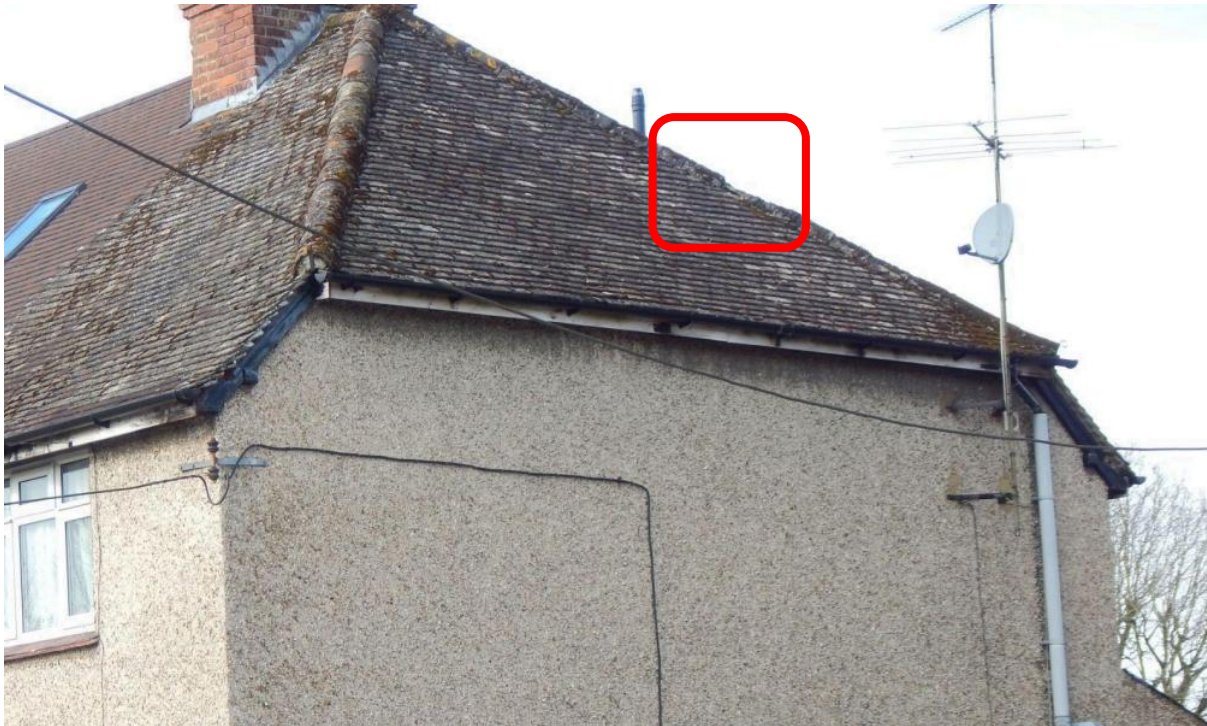
Image 5 – North facing elevation n of the property where gaps of adequate proportions to offer likely shelter/access opportunities for bats were observed within the hip coverings
