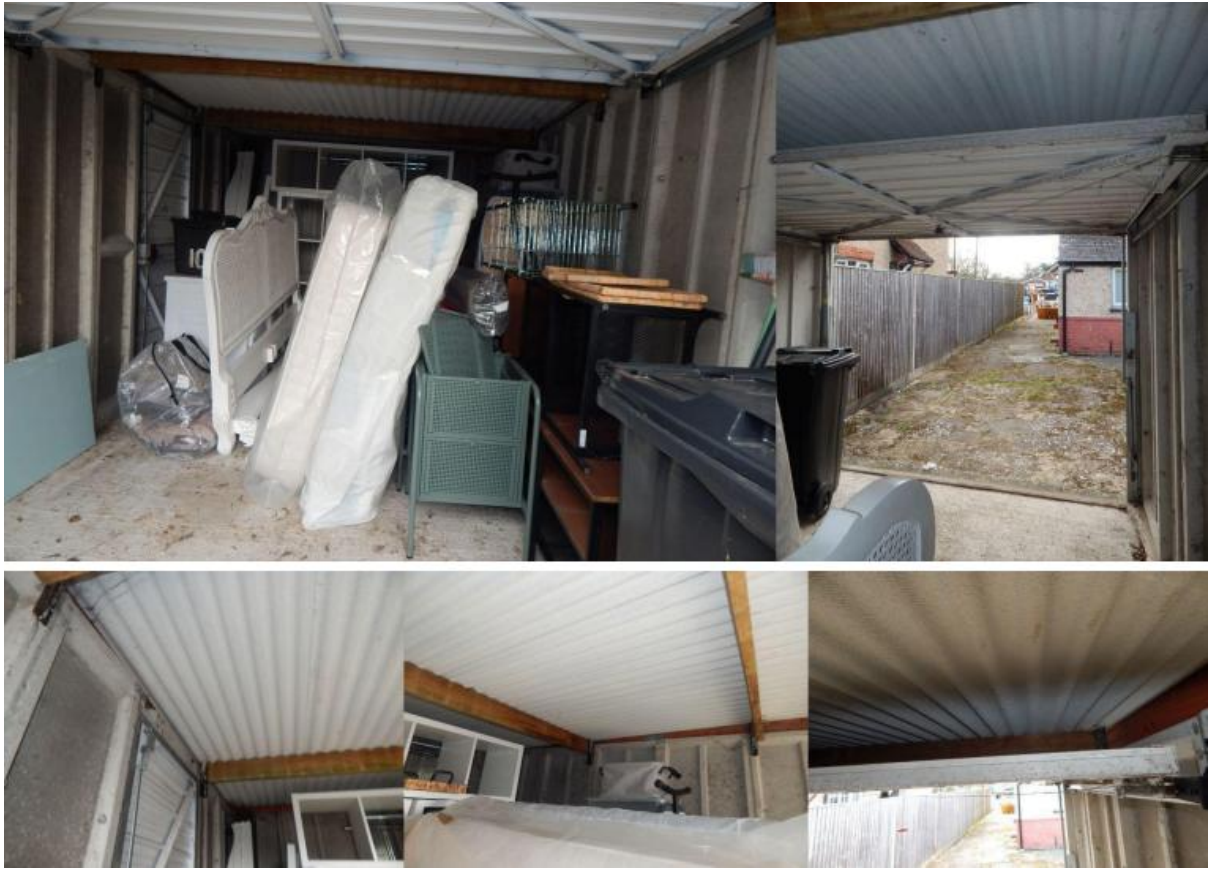
Image 9 – Internal view from within the detached garage structure
