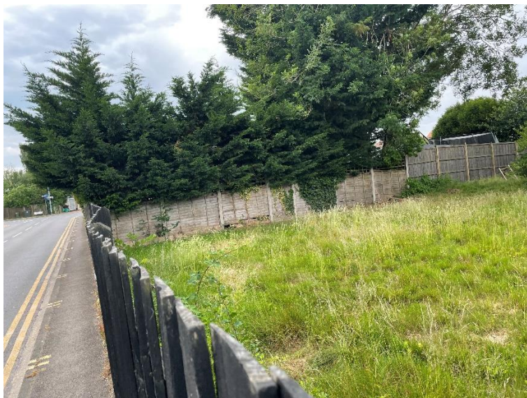
Fence on the south side of the site
