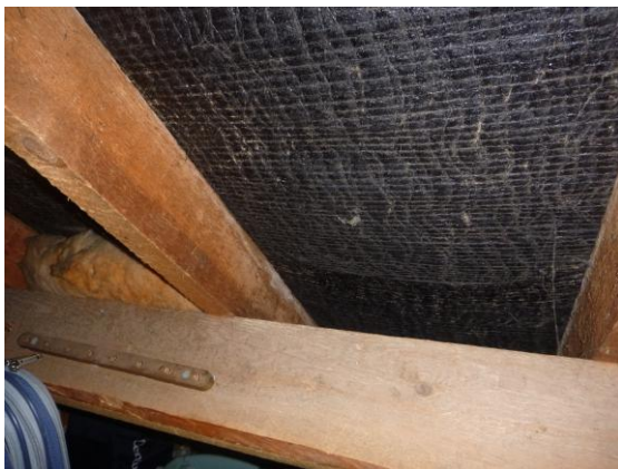
Photograph 9. Bitumen reinforced roof liner with
