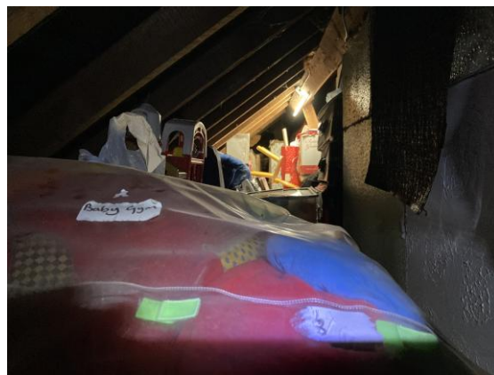
Photograph 8. Eaves space with height of approx. 1.6m.
