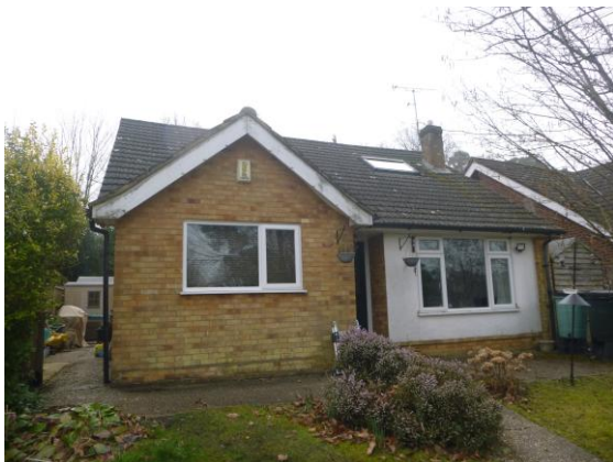
Photograph 1. Front of the property viewed from the north.
