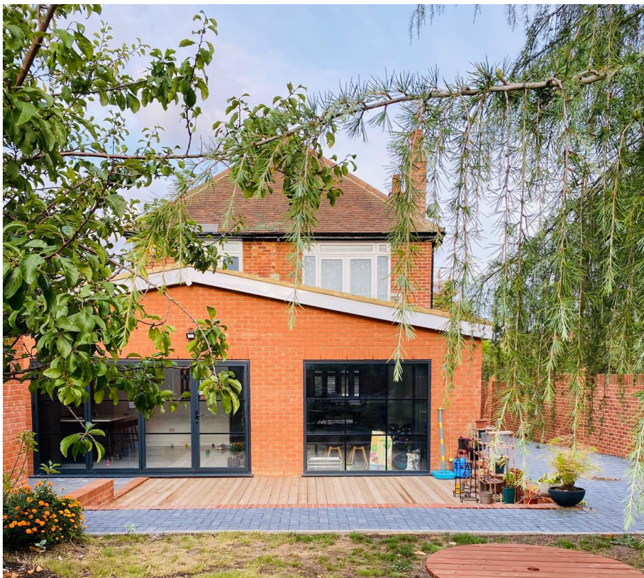
Rear Elevation of Bluehill
