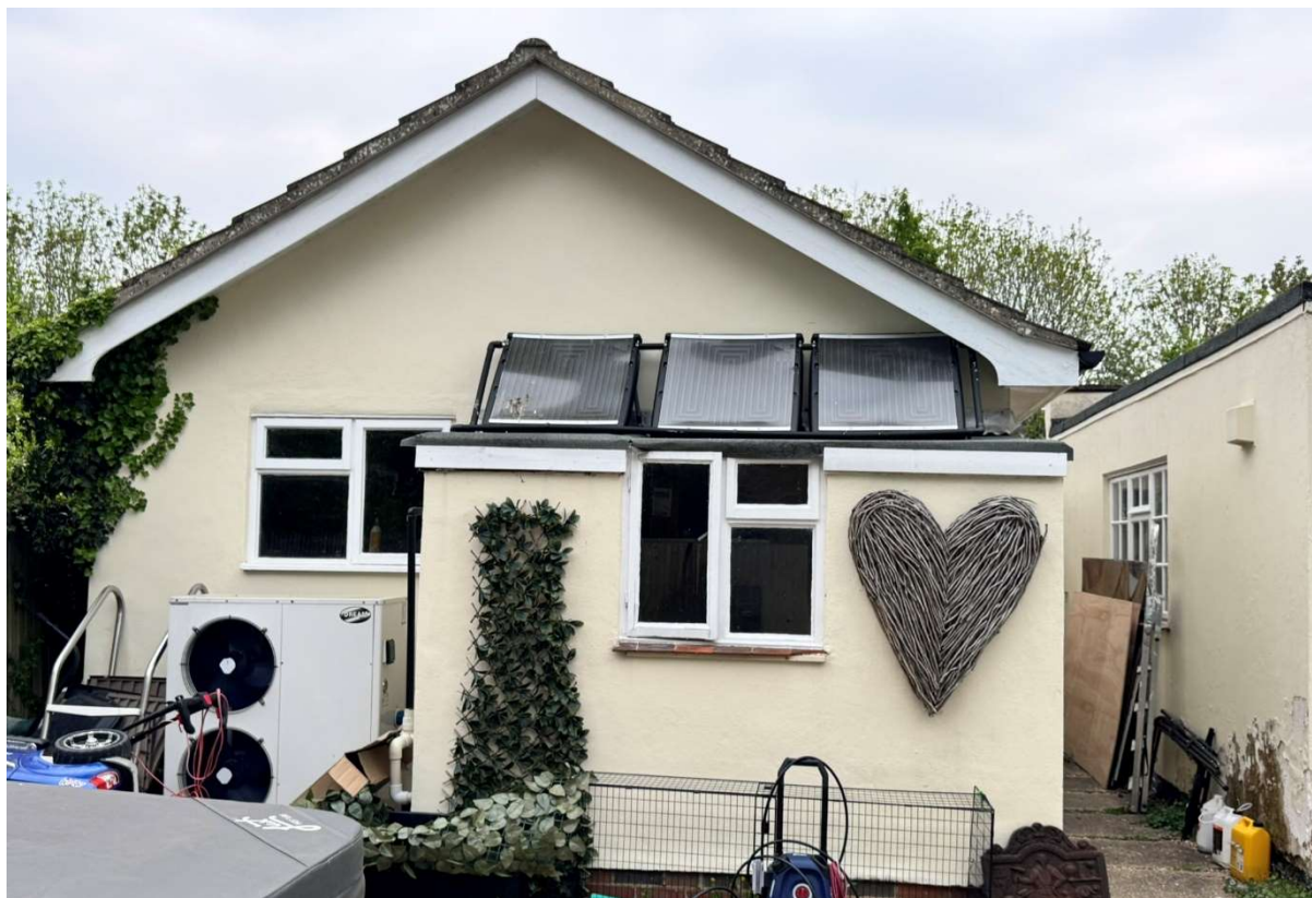
Pic. 3 – Existing Garage & Plant Room
