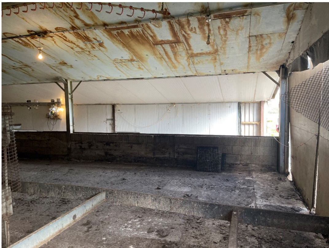
Photo 17 – Inside to rear with floor grating removed Stepped concrete floor slab exposed and found to be in good condition
