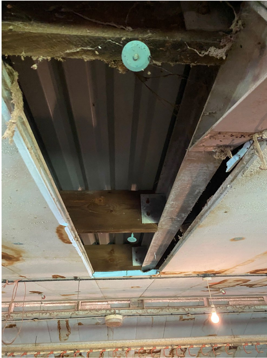
Photo 18– Portal roof rafters with timber purlins All in good condition
