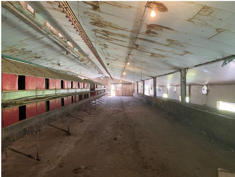
Photo 16 – Inside looking toward the rear with floor grating removed Concrete floor slab exposed and found to be in good condition
