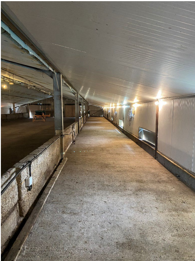
Photo 19 & 20 – Inside to rear with floor grating removed Concrete floor slab cleaned and found to be in excellent condition. No change in structural integrity of the building.
