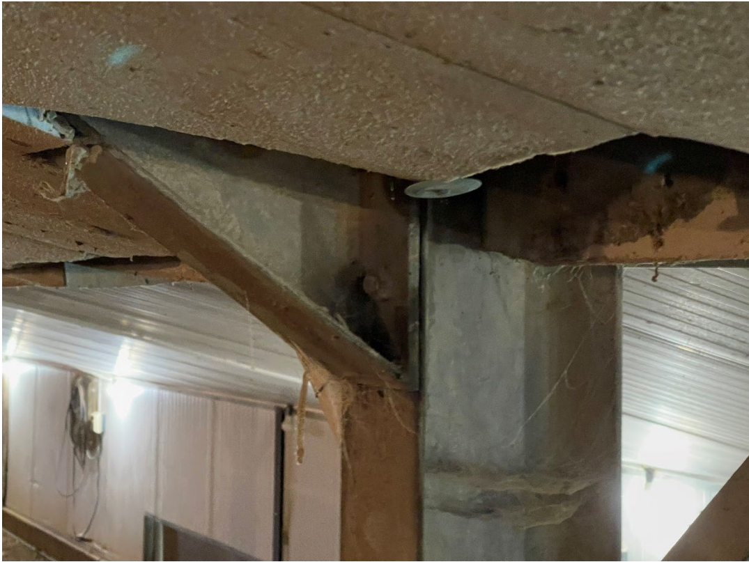
Photo 13 – Portal Column haunch detail
