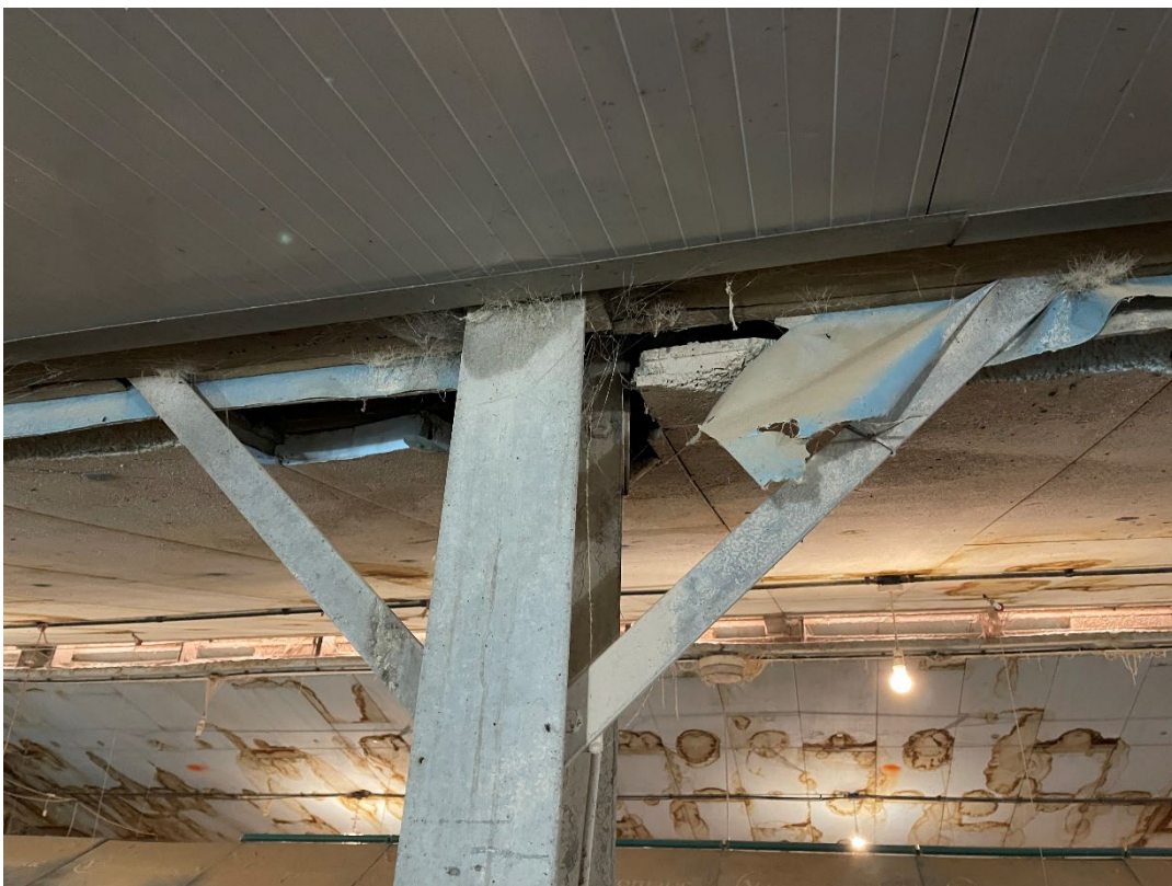
Photo 12 – Substantial Portal Column head restraint detail
