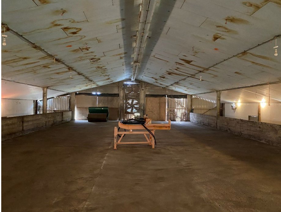
Photo 19 & 20 – Inside to rear with floor grating removed Concrete floor slab cleaned and found to be in excellent condition. No change in structural integrity of the building.
