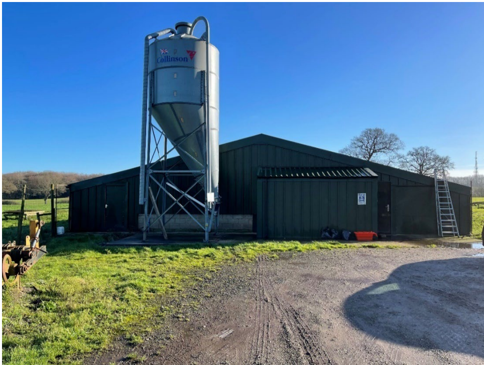
Photo 01 – Side - West Elevation
