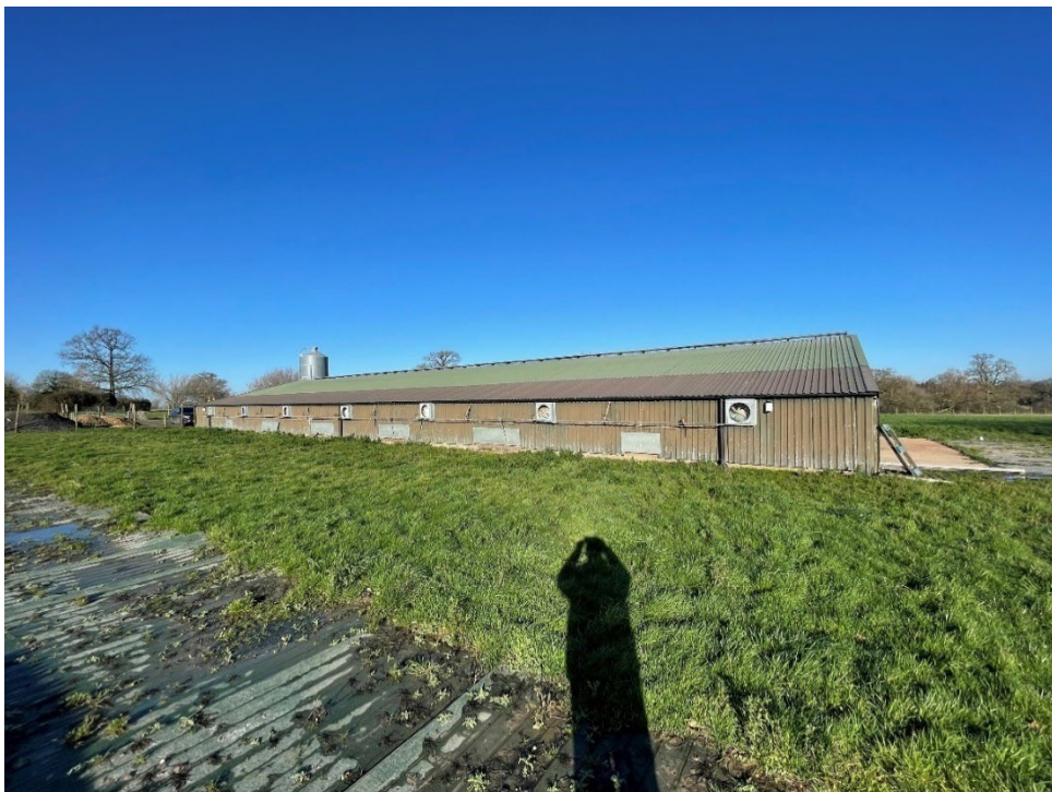
Photo 02 – Rear - South Elevation
