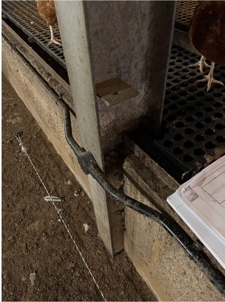
Photo 11 – Portal Column detail – showing block wall and raised floor grating
