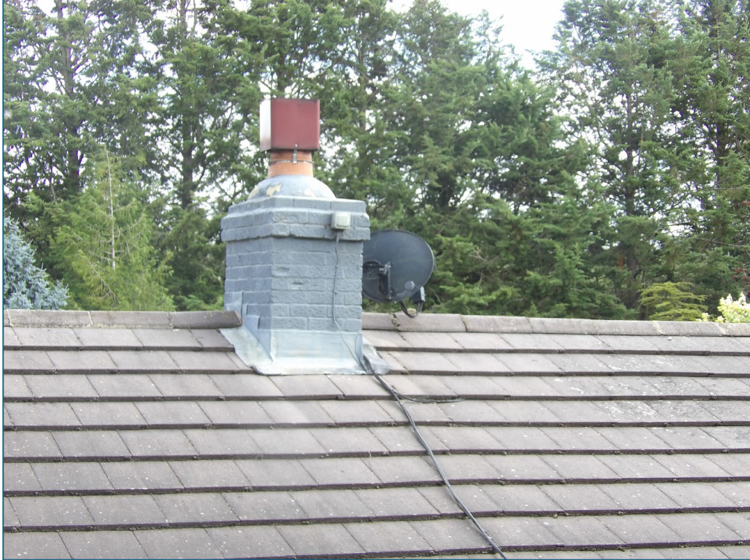
Figure 5. Example of sealed ridge tiles and lead flashing. Waters Edge, Wargrave. 05.08.25
