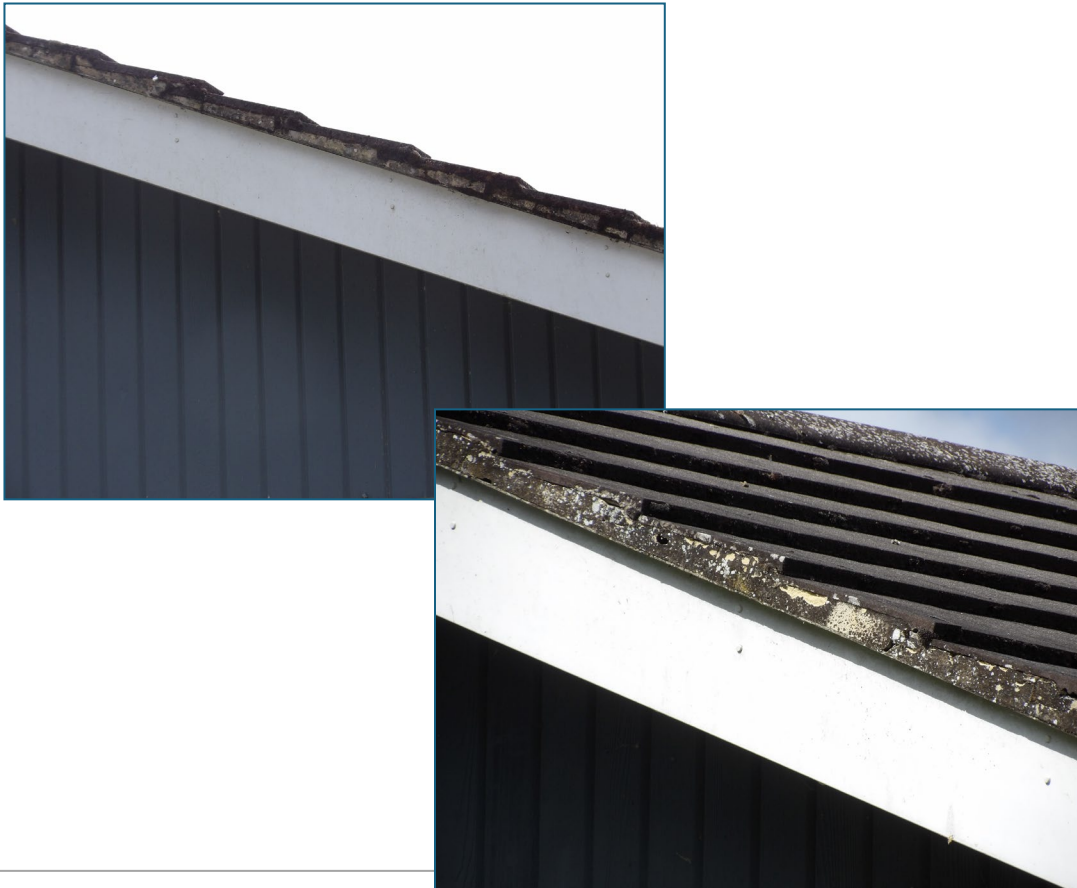
Figure 6. Example sealed verges. Waters Edge, Wargrave. 05.08.25
