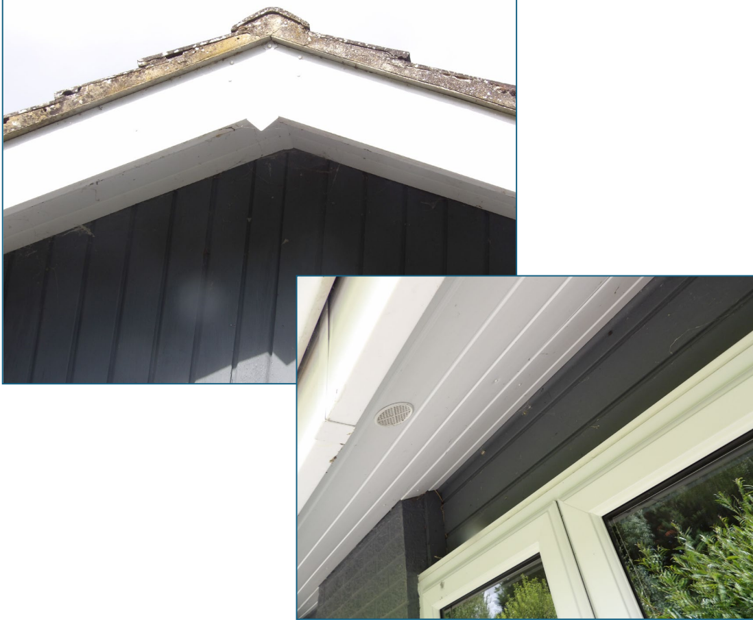
Figure 8. Example tightly fitted cladding. Waters Edge, Wargrave. 05.08.25
