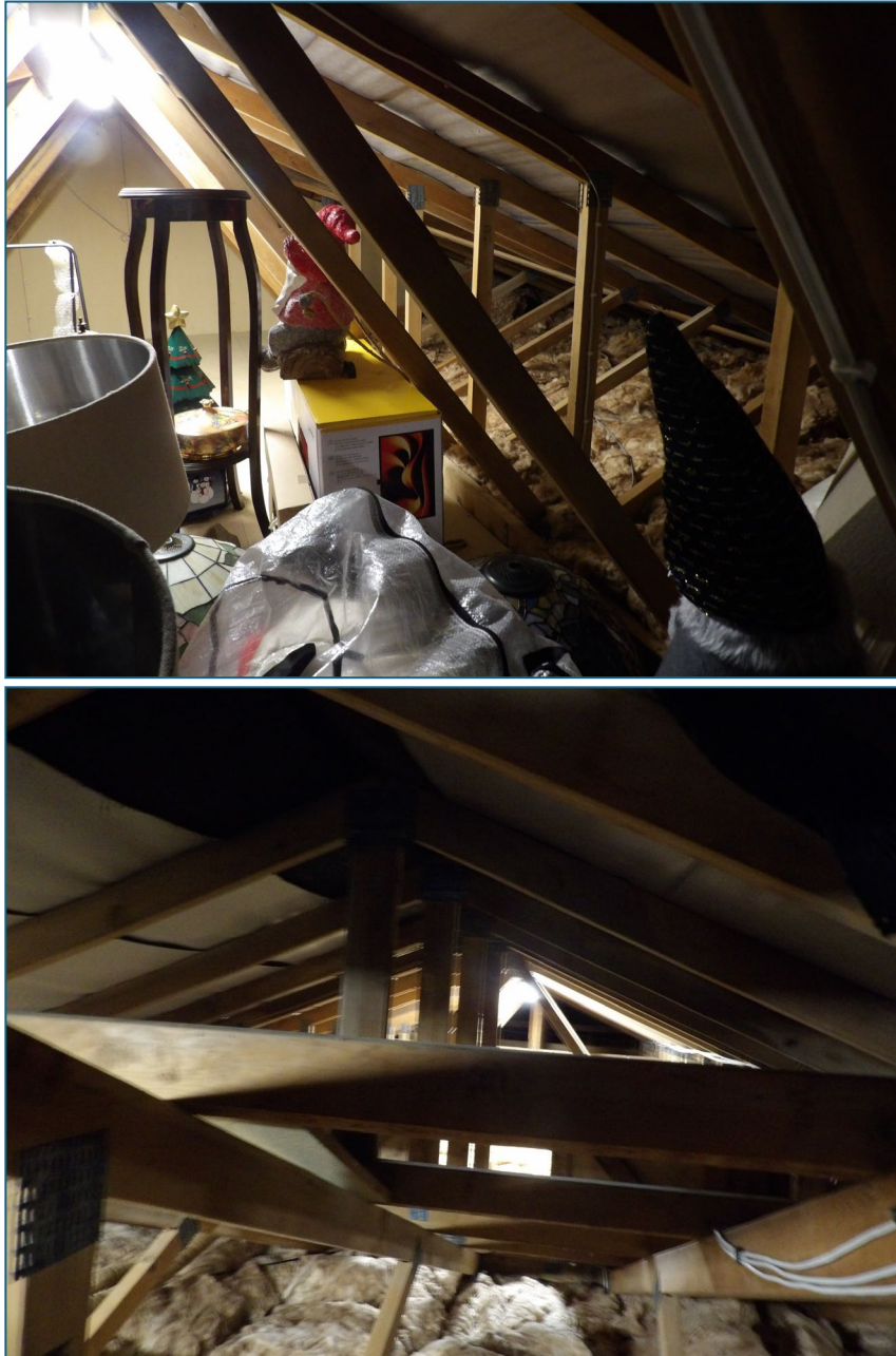
Figure 9. Example of loft space. Waters Edge, Wargrave. 05.08.25
