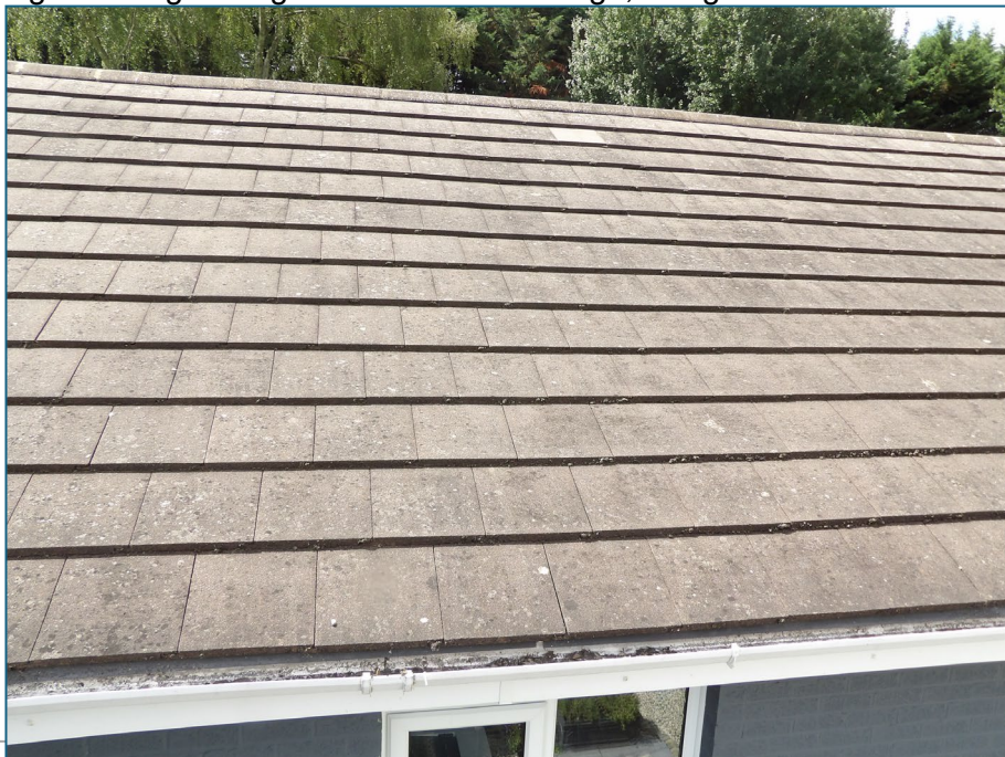
Figure 4. Tigh fitting roof tiles. Waters Edge, Wargrave. 05.08.25
