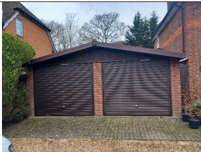
Photo 2: B1b – Southeast elevation.
