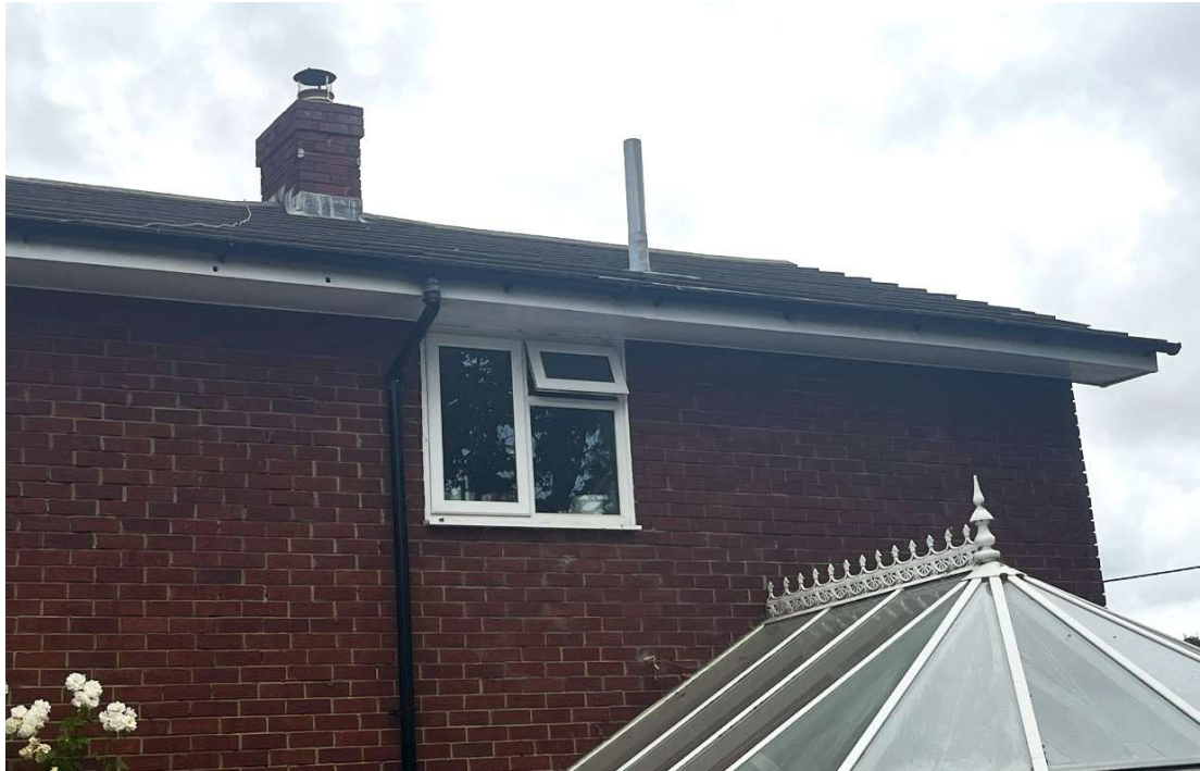
Figure 8. Eastern elevations of house and conservatory looking west
