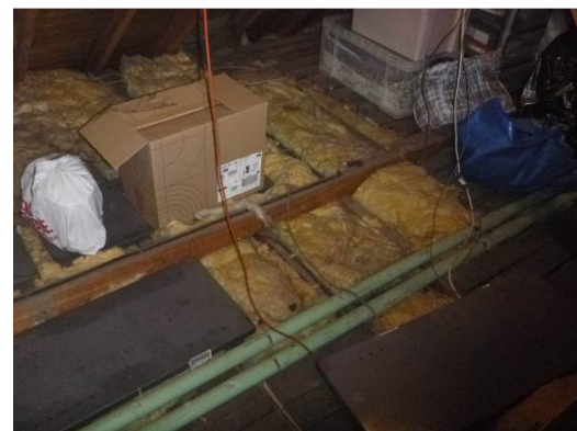
Photograph 19. Fibreglass between joists.
