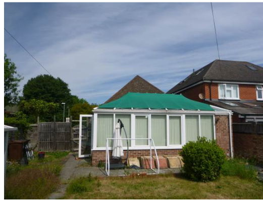
Photograph 2. Side conservatory viewed from southeast.
