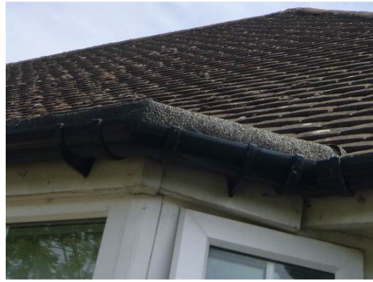
Photograph 7. Tight bitumen flat roofs (front elevation).
