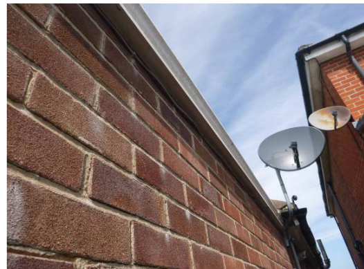
Photograph 11. uPVC of the conservatory roof tightly fitted to the brick work (south-east elevation)
