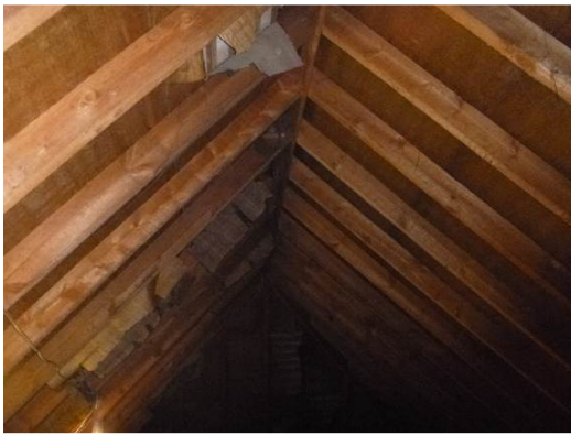
Photograph 14. Timber 'cut and pitch' roof construction with heavily cobwebbed ridge.
