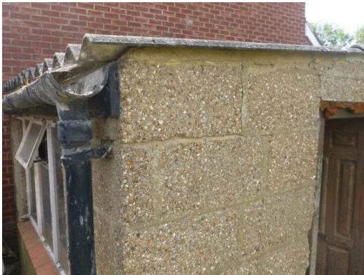
Photograph 12. Sloping corrugated asbestos roof (southeast elevation).
