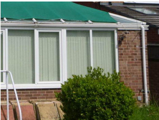
Photograph 10. Tight uPVC to brick base and side of conservatory (south elevation)
