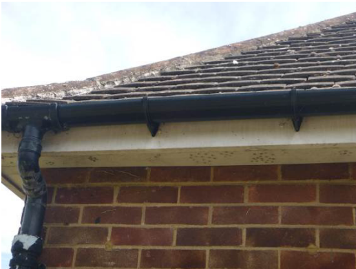
Photograph 8. Intact soffits (northwest elevation).
