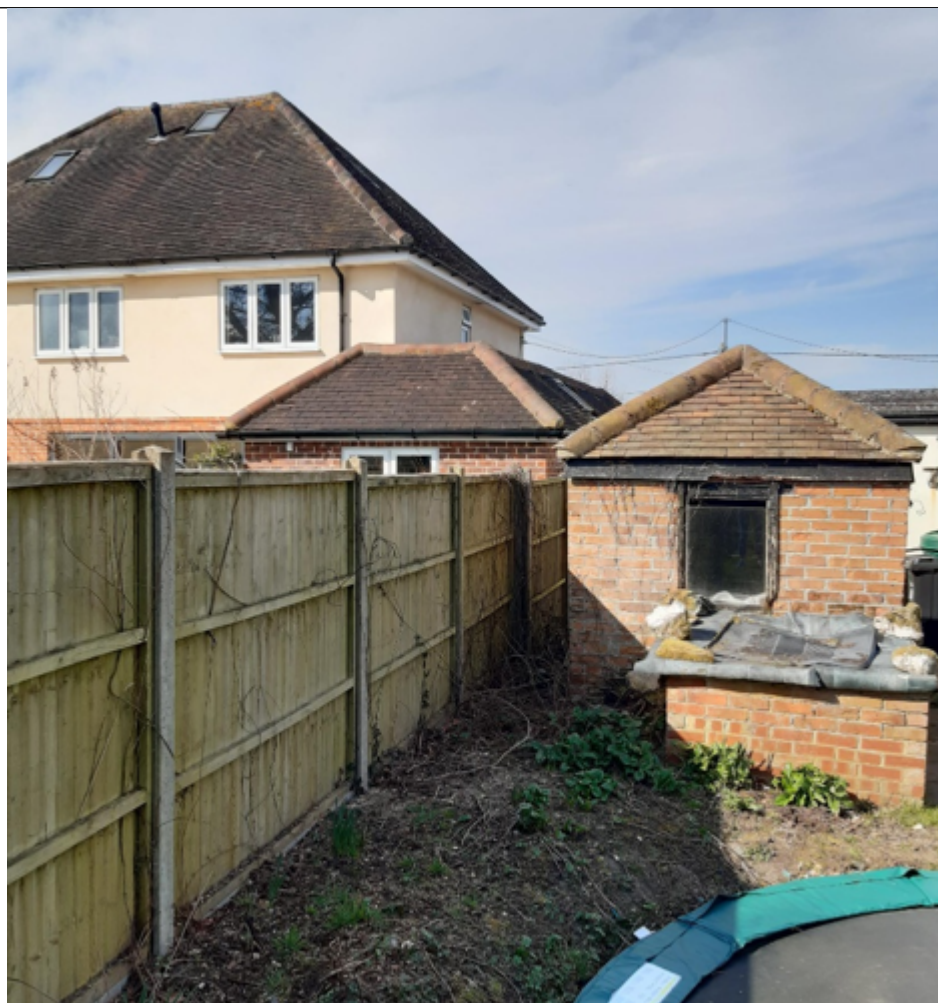
Figure 1: Existing outbuilding located along the shared boundary with no. 7.
