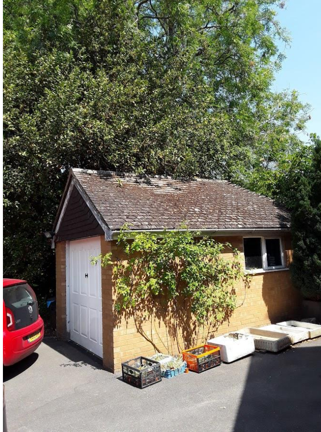
Figure 1 – Looking northwards at the existing garage to be demolished.
