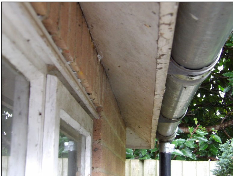
Figure 7. Example of sealed fascia. Powerscourt, Woodley. 01.10.24
