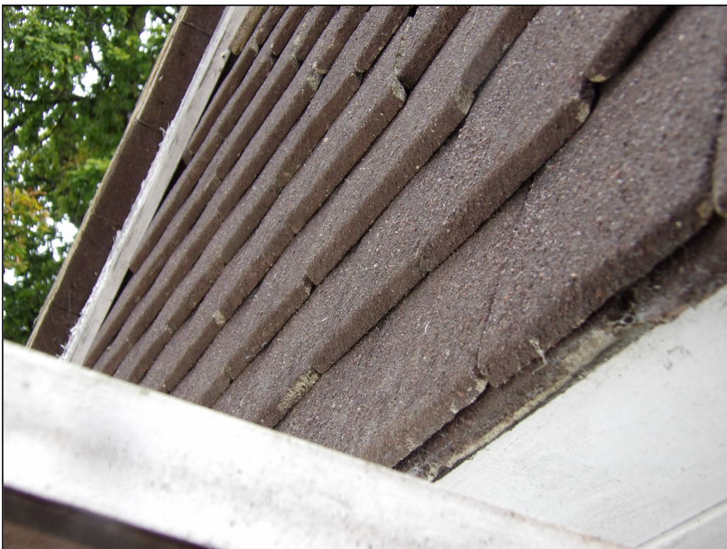
Figure 9. Example of tightly fitted hanging tiles on front elevation. Powerscourt, Woodley. 01.10.24
