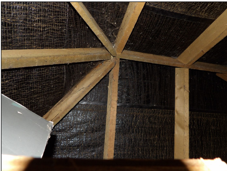
Figure 11. Bitumen lining of garage roof. Powerscourt, Woodley. 01.10.24
