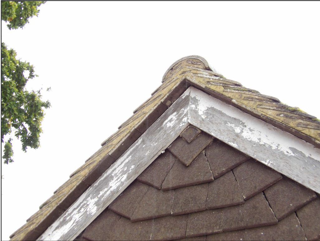
Figure 8. Example of sealed verges. Powerscourt, Woodley. 01.10.24
