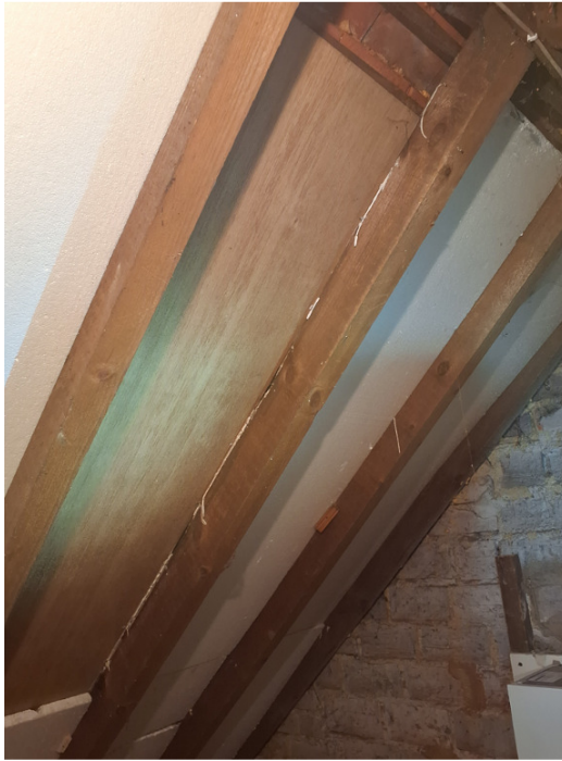
Photograph 10. Timber boarding behind polystyrene.
