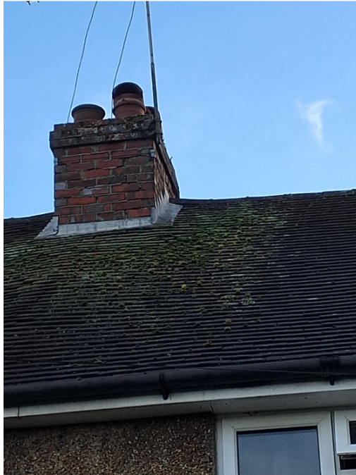
Photograph 5. Raised ridge tile against the chimney (front elevation).
