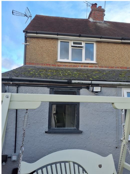
Photograph 8. Slate tiles fully sealed (rear elevation).
