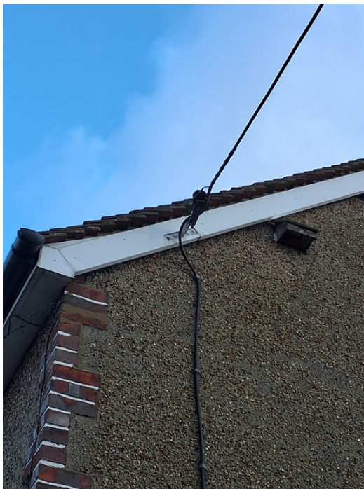
Photograph 3. Verge mortar fully intact along the gable (west elevation).
