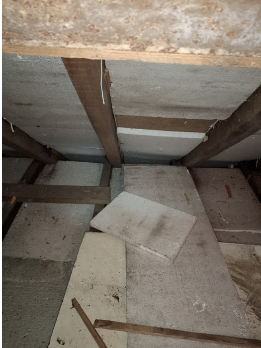
Photograph 12. Open eaves with access to the uPVC soffit.
