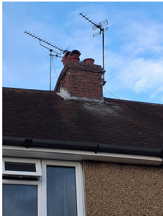
Photograph 4. Lead flashing sealed to brickwork chimney and roof tiles (rear elevation).
