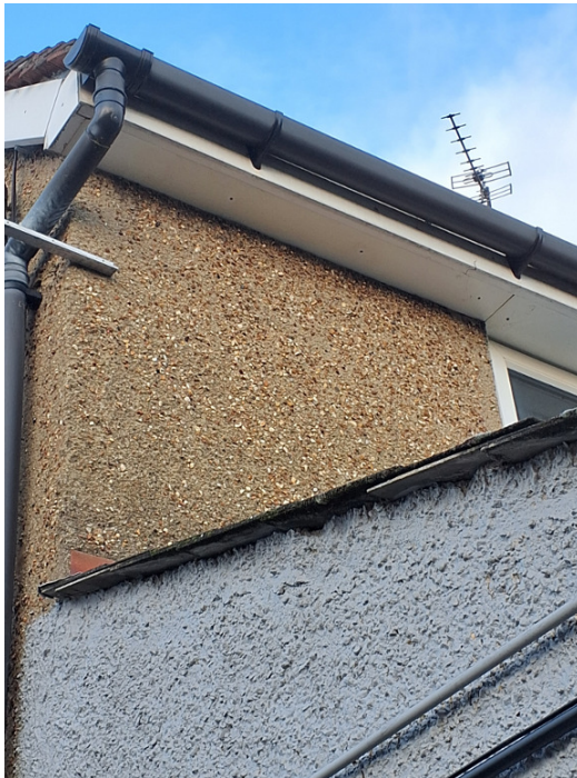
Photograph 6. uPVC soffit sealed to pebbledash wall (rear elevation).
