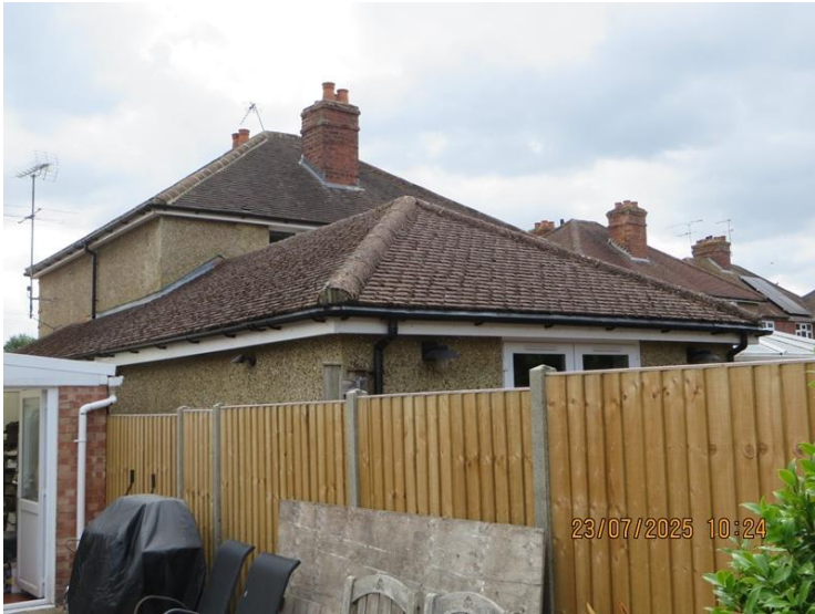
Rear elevation neighbouring 203 Loddon Bridge Road
