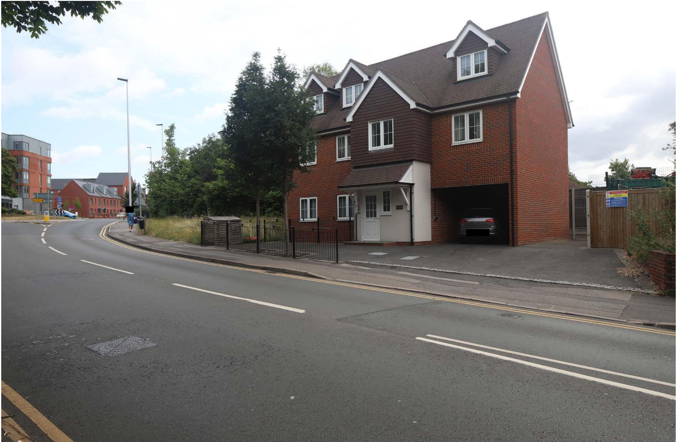
Representative View 2 - Existing view
