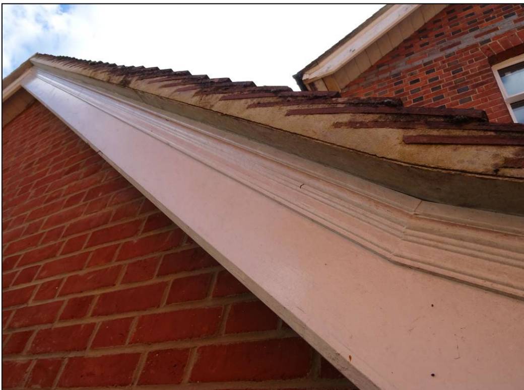
Figure 7. Example of verges. Westdene, Basingstoke Road, Reading. 25.04.23
