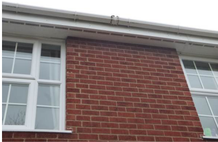
Photograph 7. Flush soffit box at eaves (front elevation).
