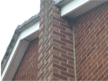
Photograph 5. Gable soffits flush to brickwork (south-western elevation).
