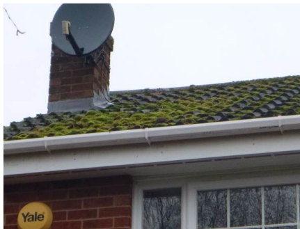
Photograph 4. Tight lead flashing around chimney (front elevation).
