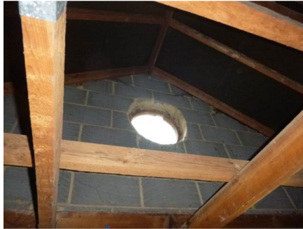
Photograph 19. Porthole window in gable wall (garage space).
