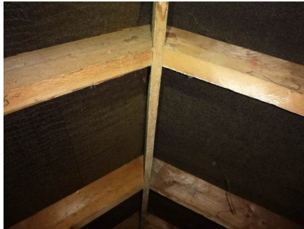
Photograph 12. Intact bituminous roof lining (roof void).
