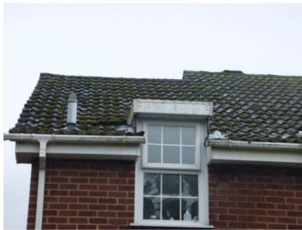
Photograph 8. Dormer window on rear catslide (rear elevation).
