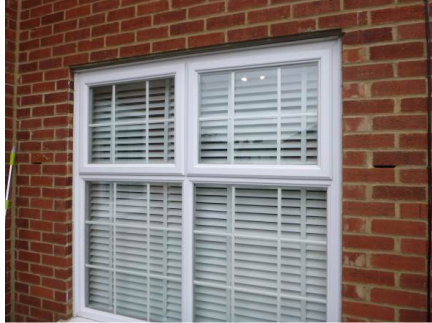
Photograph 10. Weeps holes either side of window (front elevation).
