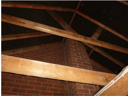
Photograph 18. Garage space open to rafters.
