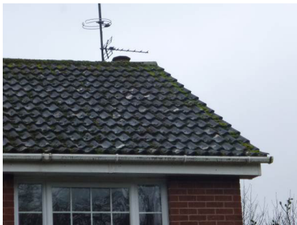
Photograph 3. Tight interlocking roof tiles with fully mortared ridge (front elevation).
