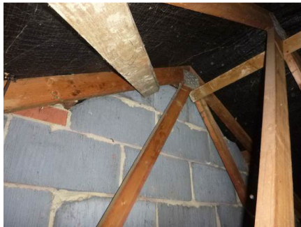
Photograph 17. South-western gable end (roof void).
