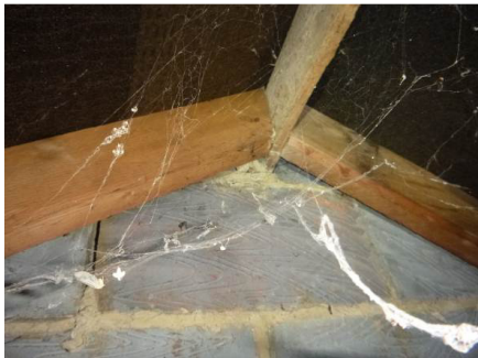
Photograph 16. Side extension gable end (roof void).
