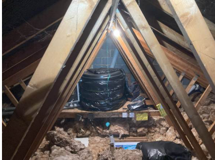
Photograph 14. Covered water tank (roof void).
