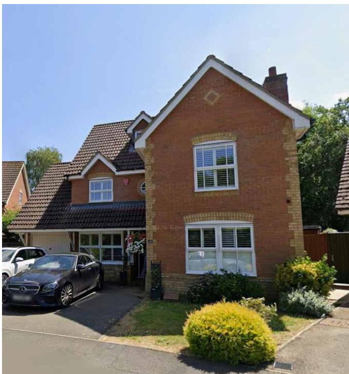
Flush quoining, detail in the gable, double brick arch headers
