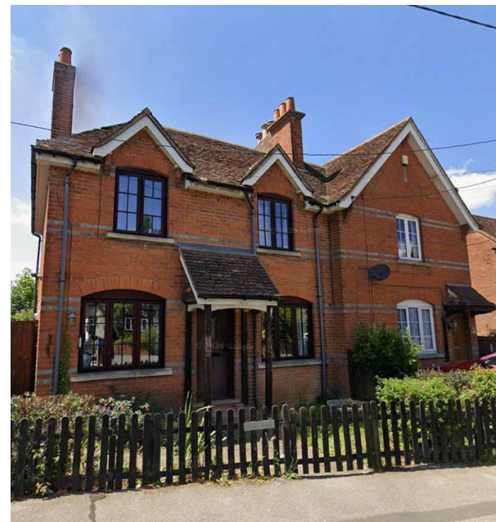
Flush banding with a dark brick
