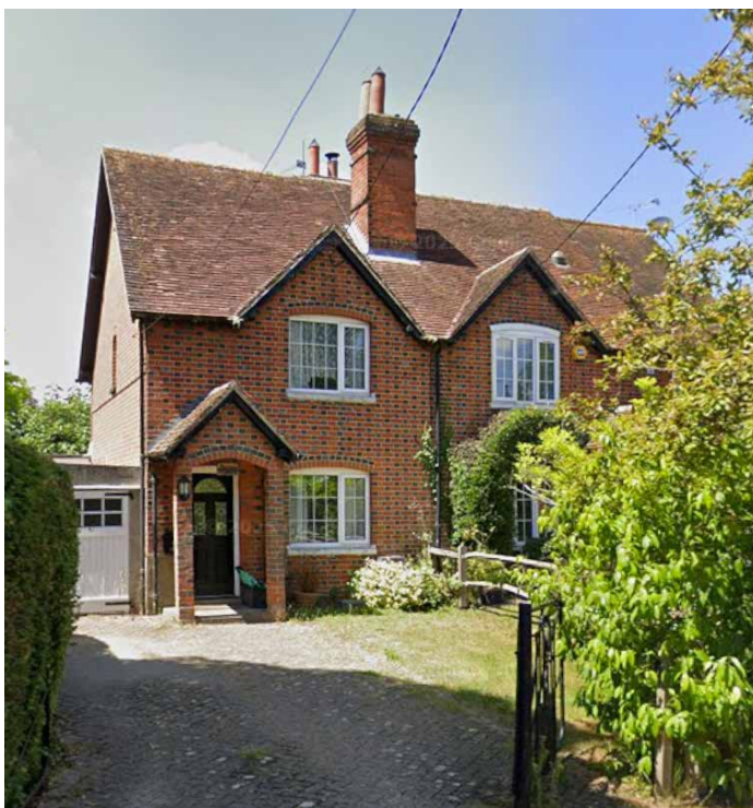
Flemish bond with burnt headers
