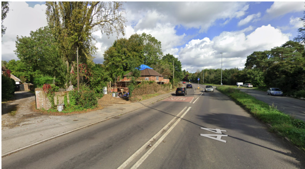
VIEW OF ENTRANCE DURING CONSTRUCTION
